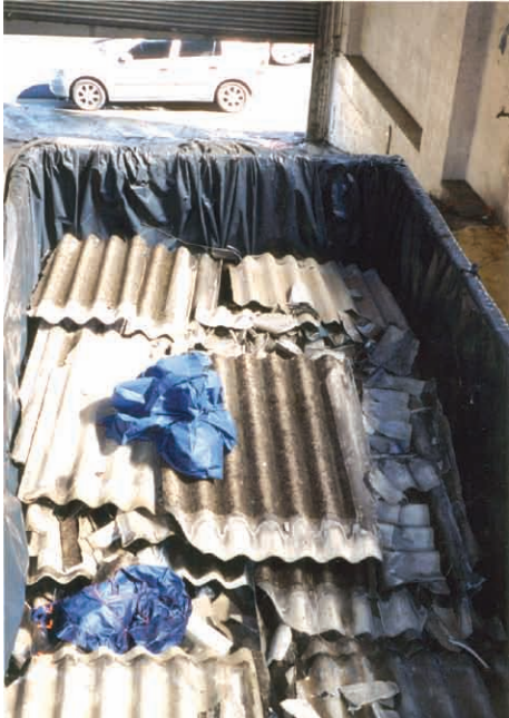
LINING BINS IN 200micron PLASTIC
