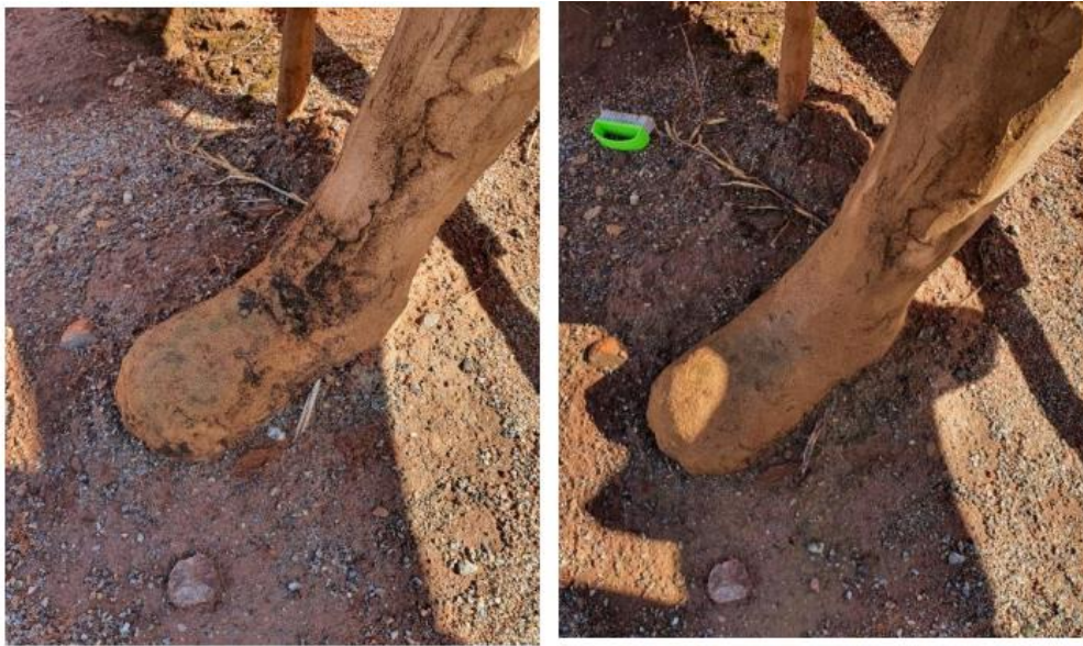
Figure 62-63 Detail biological growth – Before and after cleaning with biocide.
