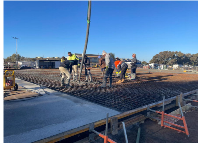
Final placement of concrete slab – 23 July 25
