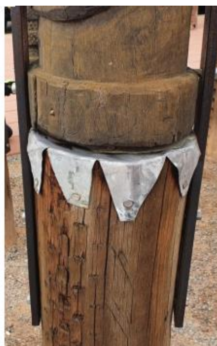
Figure 57 Detail – Metal corrosion products after intervention.
