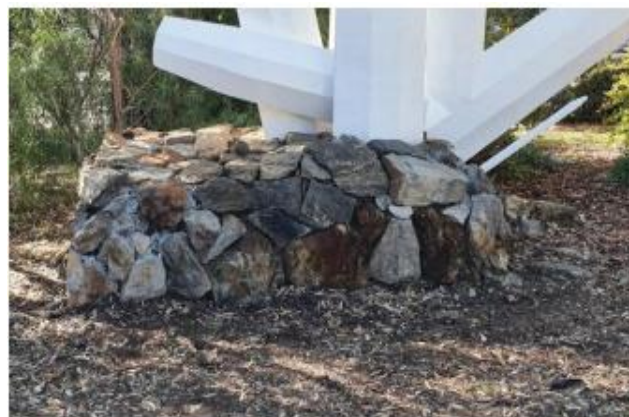
Figure 6 Plinth – After stone relocation and stabilization.
