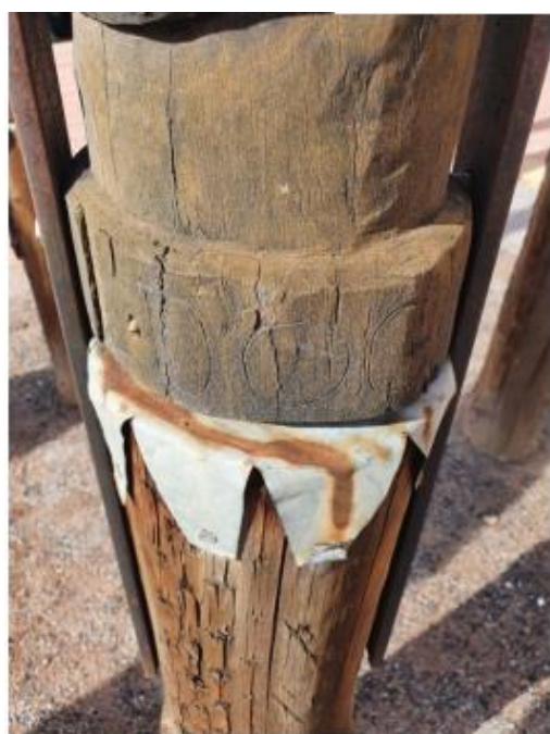
Figure 567 Detail – Metal corrosion products before intervention.
