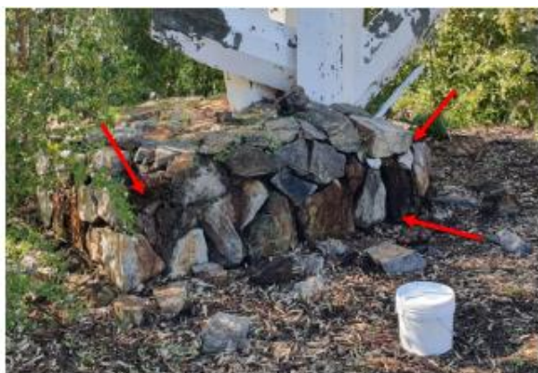
Figure 5 Plinth – Before re-pointing and stone relocation (in red).
