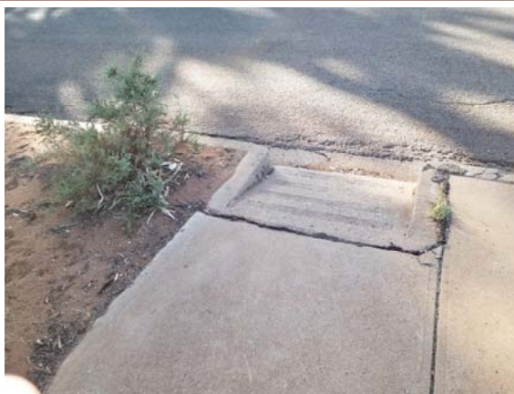
Figure 8-21 Wolfram Street - Non-compliant kerb ramp
