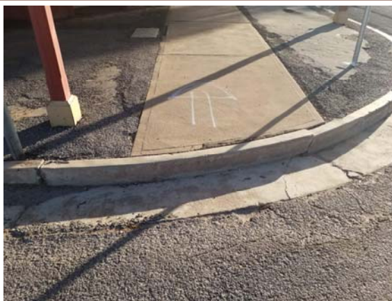
Figure 8-21 Wolfram Street - Non-compliant kerb ramp
