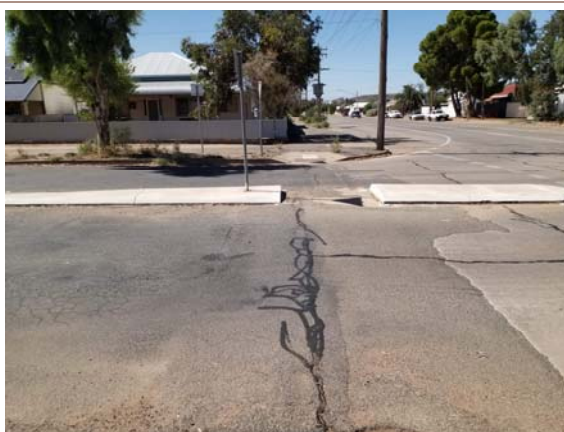
Figure 8-25 Chapple Street - Non-compliant pedestrian refuge
