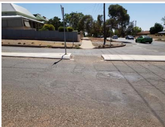
Figure 8-25 Chapple Street - Non-compliant pedestrian refuge
