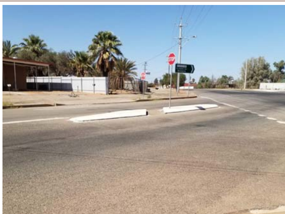
Figure 8-24 Williams Street - Non-compliant pedestrian refuge
