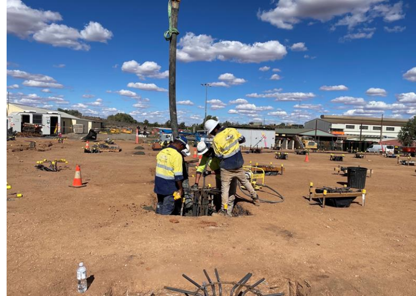
Placement of Piles on site – 24 April 2025
