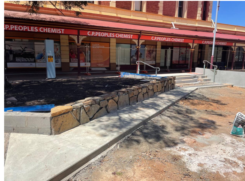
Low level garden wall – stone works underway in January 2025
