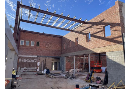
1 st Roof Steel Modules – 28 April
