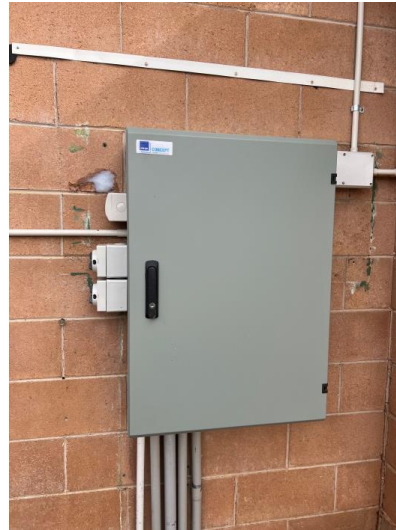
Images: Upgraded switchboard
