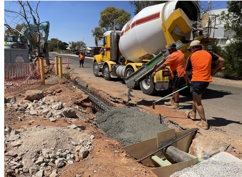
Concrete pipe encasement (shallow depths) – March 2025
