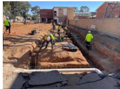
Image right: Steel fixers working on preparing footings
