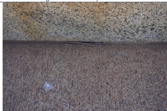
Figure 20: Detail – loss to mortar pointing and bird excrement.
