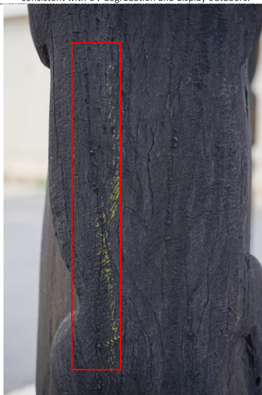
Figure 123: Detail – Pole #2003.0026, Reconciliation , exterior, UV degradation (darkening) to wood surface throughout. A large linear accretion, yellow in colour (highlighted in red), is present on the exterior side of the pole.
