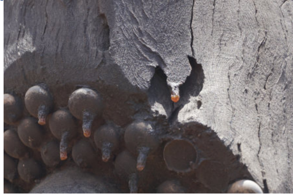
Detail 70: Detail – Pole 9, exterior, UV degradation (darkening) to wood surface, sap-like deposits (accretions) above the carved figure surrounded by glass pebbles.
