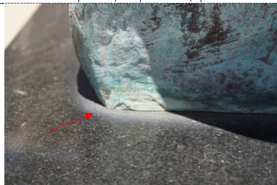
Figure 14: Detail – increased copper corrosion product stemming from collected water at plinth interface.
