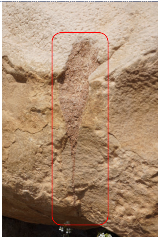
Figure 11: Detail – mortar fill.
