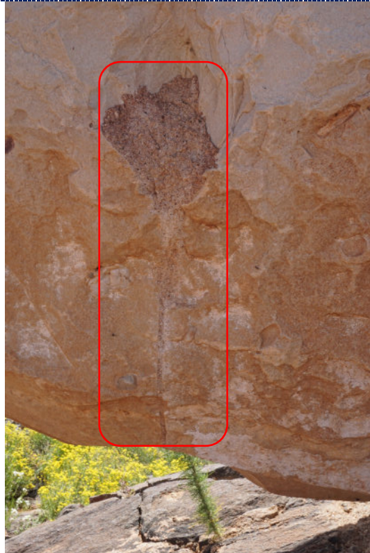
Figure 14: Detail – mortar fill.
