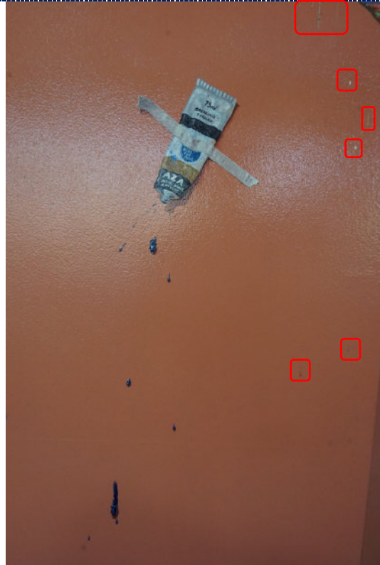
Figure 30: Work 14 – Detail – Surface accretions.
