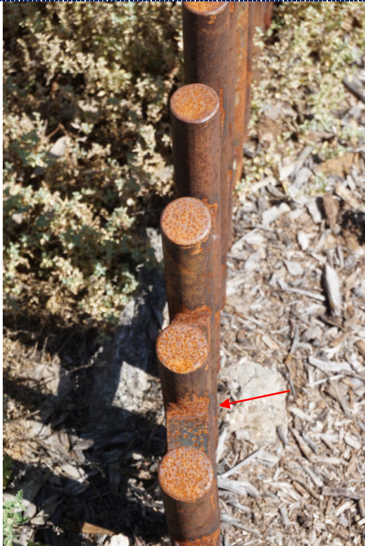
Figure 9: Detail – dirt particulate; surface flash rusting at new welds created during manufacture of artwork.
