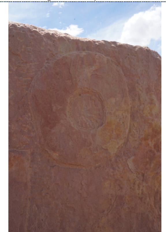
Figure 10: Detail – possible surface delamination.
