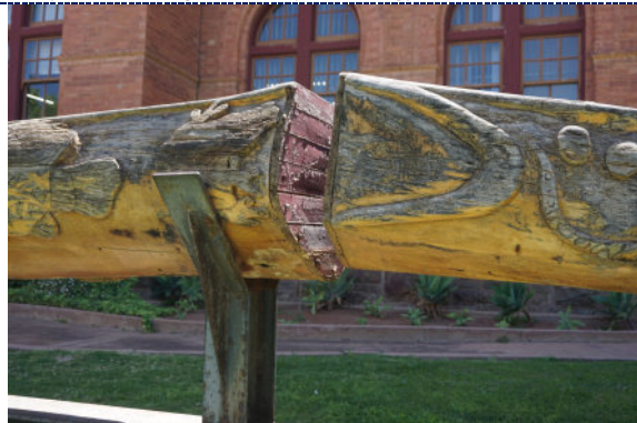
Figure 23: Detail – exterior, degraded and peeling varnish, UV degradation (darkening) to wood surface, degraded and peeling maroon paint. Corrosion on mount.
