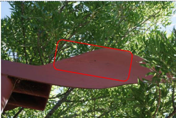
Figure 5: Detail – flaking paint loss.
