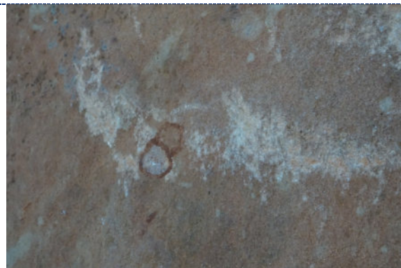
Figure 10: Detail – figure "8" inscription/accretion noted.
