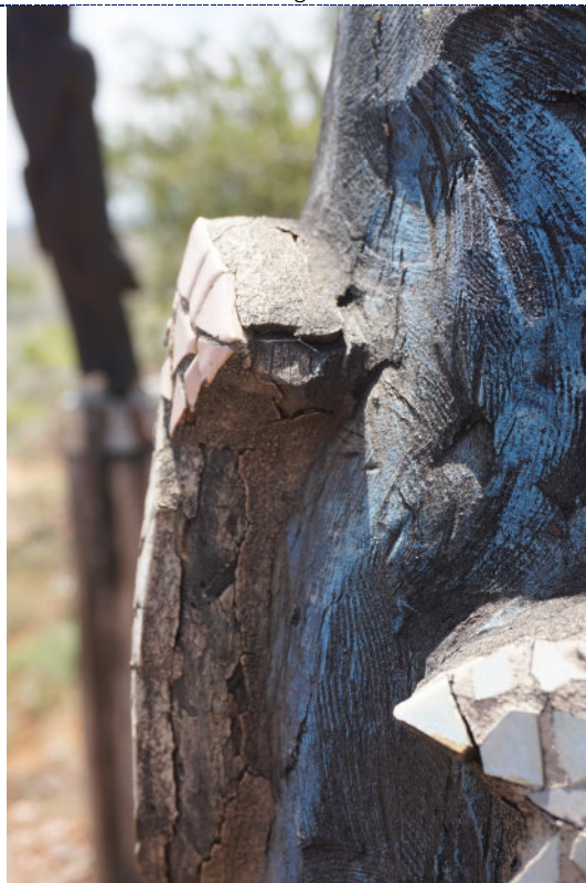
Figure 57: Detail – Pole 8, exterior, UV degradation (darkening) to wood surface, extensive losses to wood and painted surfaces and degradation to the binder securing the mosaic tiles in place.
