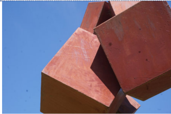
Figure 5: Detail – paint chalking, flaking paint loss with overpaint.
