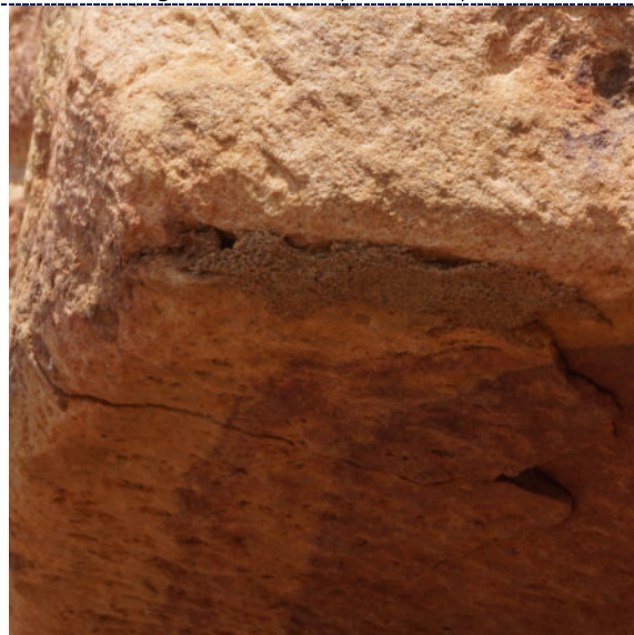
Figure 14: Detail – verso upper, previous repair.
