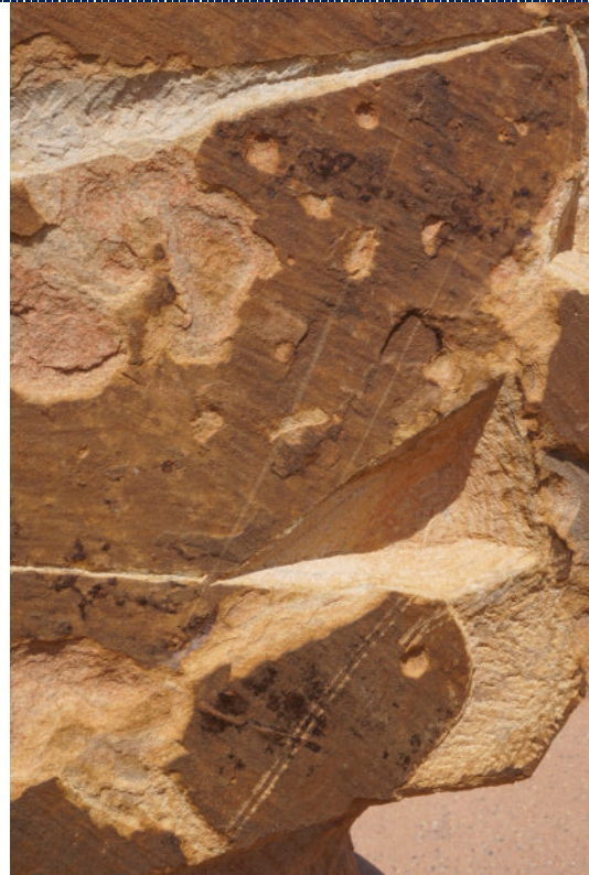
Figure 6: Details – surface abrasions and delamination.
