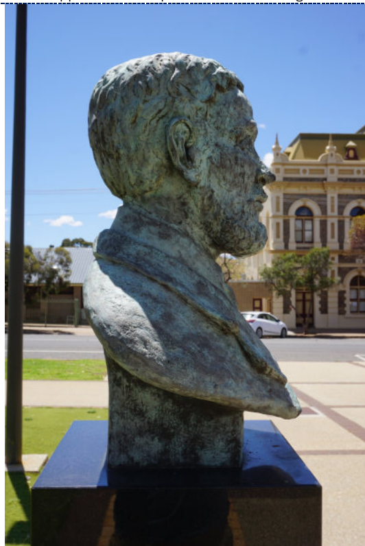
Figure 8: Detail – bust, proper right. Atmospheric pollution-driven copper corrosion product on bronze figure.
