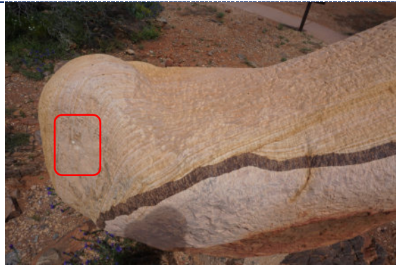
Figure 13: Detail – white accretion, possibly an unknown paint polymer.
