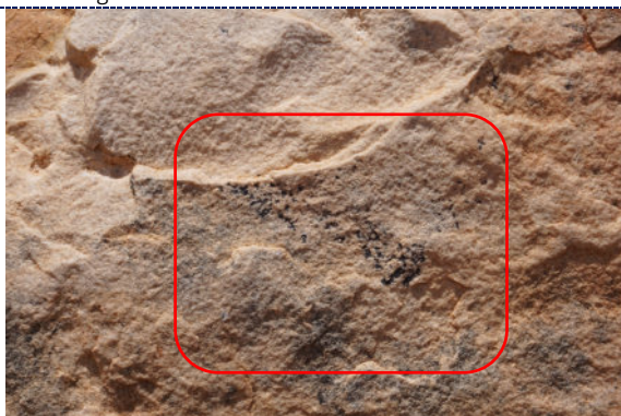
Figure 11: Detail – unknown surface accretion.
