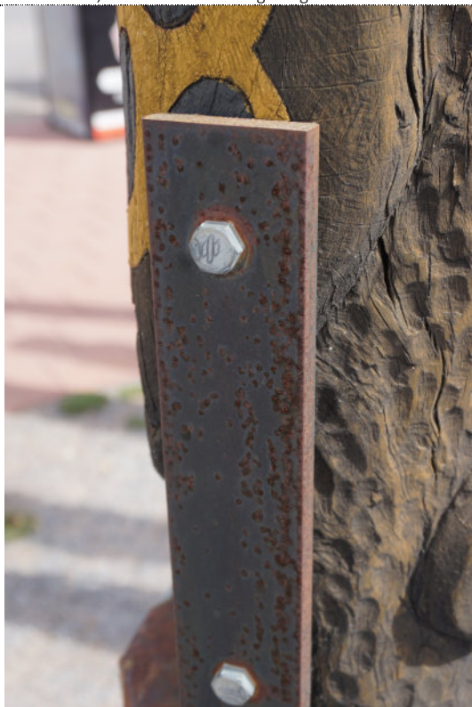
Figure 25: Detail – Pole #2003.0018 Emus and eggs , exterior, extensive corrosion products on iron structural support, UV degradation (darkening) to wood surface, and extensive fine cracks along the grain of the wood.
