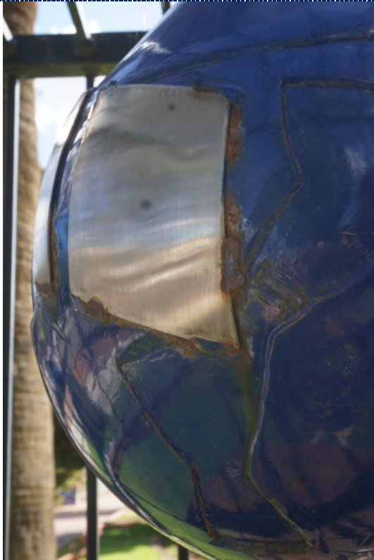
Figure 9: Detail – steel plate on surface of 'drop' (unclear if original or not). Extensive corrosion of welds surrounding the plate
