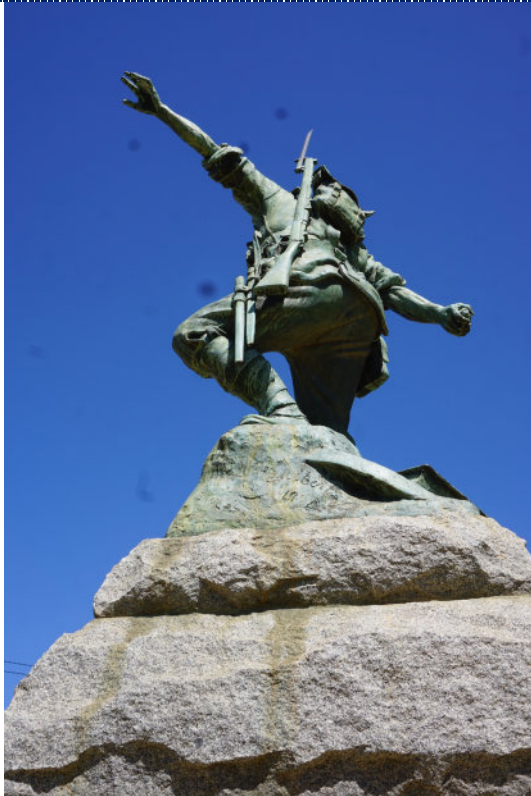
Figure 5: Detail – copper corrosion product and staining to the granite components.
