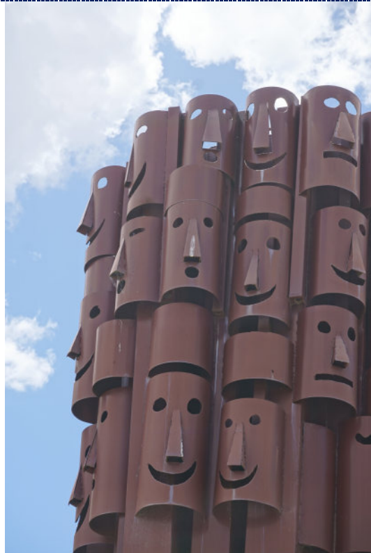
Figure 18: Detail – paint fading and degradation; dirt particulate and bird excrement.
