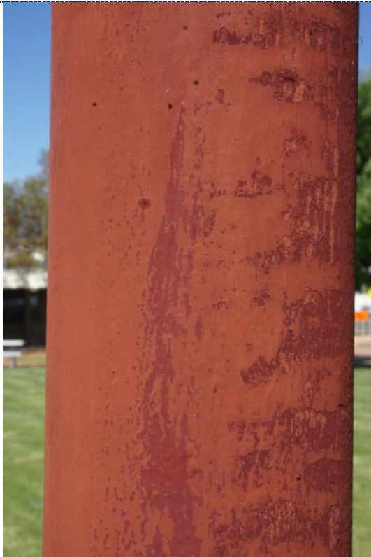
Figure 13: Detail – paint chalking. The two shades of red paint suggest the surface was repainted.
