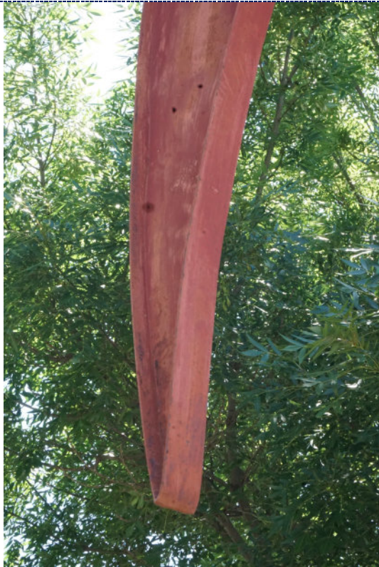
Figure 8: Detail – chalking paint, flaking paint loss, abrasions and corrosion; overpaint.
