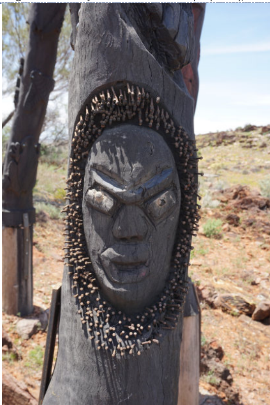
Figure 61: Detail – Pole 9, exterior, UV degradation (darkening) to wood surface, extensive losses to painted surface on carved figure’s eyes. Missing nails noted below and along the periphery of the central figure.
