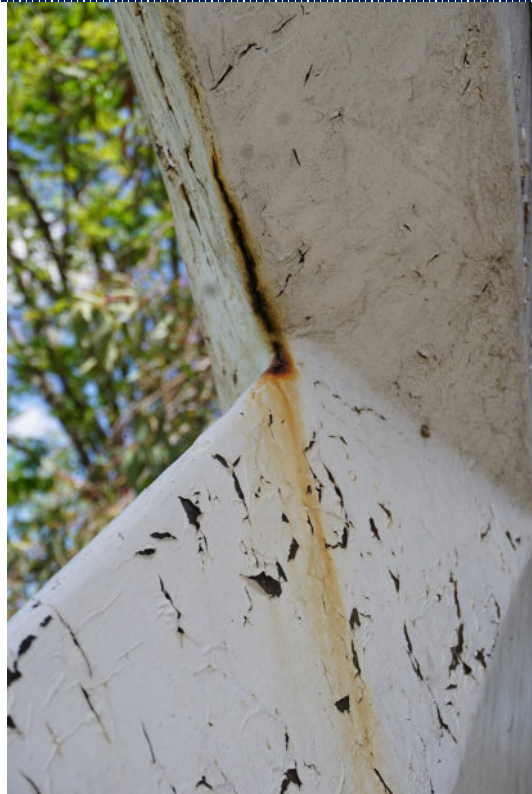
Figure 6: Detail – surface paint loss, crazing and iron corrosion product staining.
