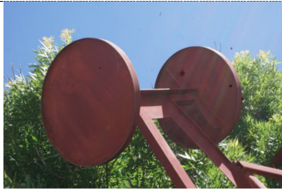
Figure 13: Detail – paint chalking, flaking, overpaint.
