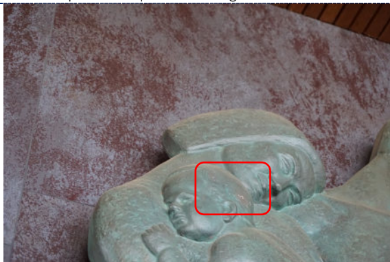
Figure 7: Detail – surface accretion, likely white paint spray.
