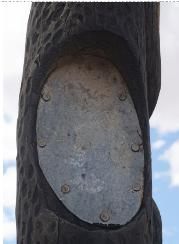
Figure 26: Detail – Pole #2003.0018 Emus and eggs , exterior, tarnishing and corrosion noted on the circular metal decorative element and nails affixing the element in place.
