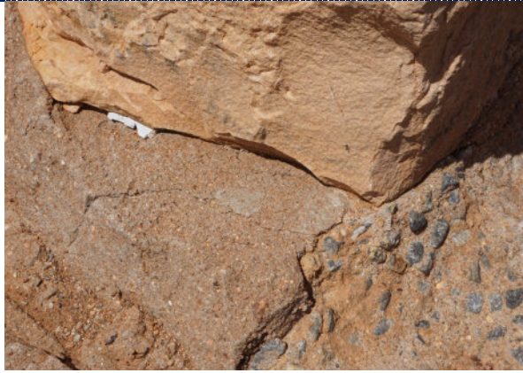
Figure 17: Detail – concrete base.
