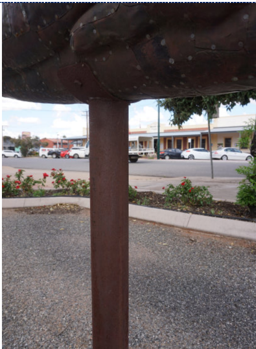
Figure 27: Detail – exterior, surface corrosion on iron mount.
