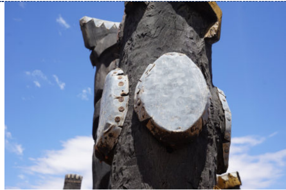
Figure 40: Detail – Pole 6, exterior, UV degradation (darkening) to wood surface, degradation of metal and presence of iron corrosion products on metal components and iron nails.
