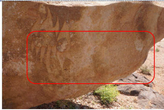
Figure 7: Detail – horizontal crack running through the rear proper right side.
