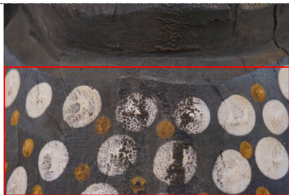
Figure 75: Detail – Pole #2003. 0022, Untitled , exterior, UV degradation (darkening) to wood surface throughout. Surface dirt also noted throughout. Fading and losses noted to the painted surfaces, particularly the white and yellow ochre painted dots (highlighted in red).
