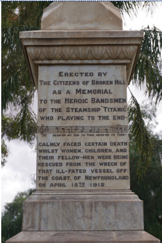
Figure 5: Detail – front, dirt particulate and stone discolouration.
