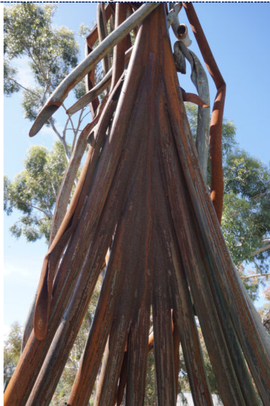
Figure 4: Detail – surface corrosion.
