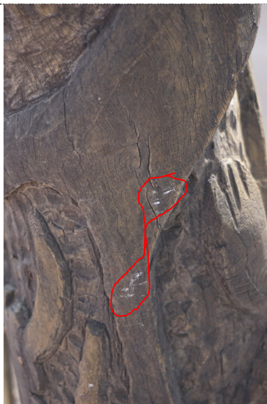
Figure 67: Detail – Pole #2003.0021 Untitled , exterior, UV degradation (darkening) to wood surface throughout. Surface dirt and insect debris noted throughout, including the presence of bird excrement (highlighted in red).
