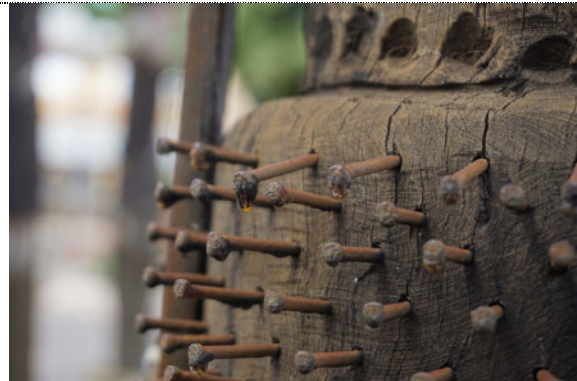
Figure 12: Detail – Pole #2003.0017 Reconciliation , proper right exterior, corroded iron nails, sap-like accretions on the iron nails, UV degradation (darkening) to wood surface, and cracks along the grain of the wood.
