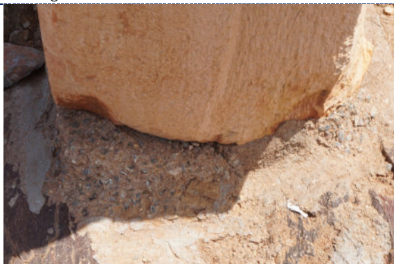
Figure 15: Detail – concrete base.
