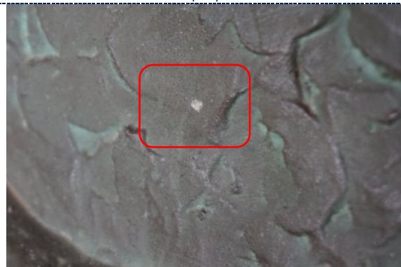
Figure 10: Detail – surface accretion, likely white paint spray.
