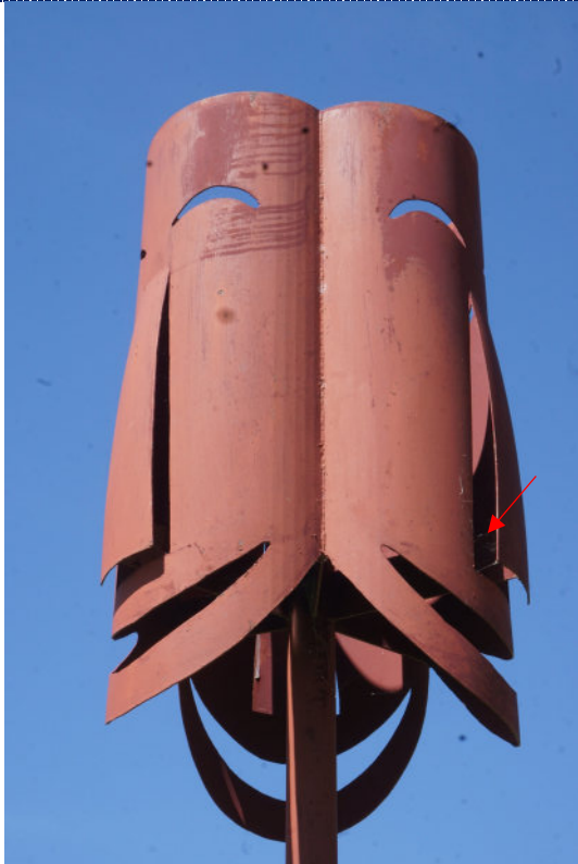
Figure 9: Detail – paint chalking, overpaint; spider webs.
