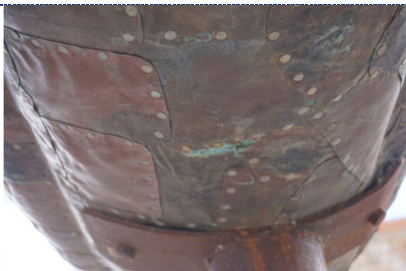
Figure 33: Detail – exterior, copper corrosion product.
