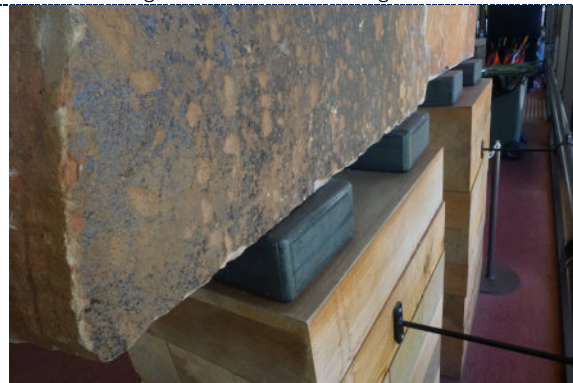
Figure 14: Detail – tidelines on timber, indicating previous exposure to moisture.
