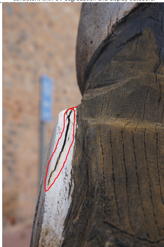
Figure 105: Detail – Pole #2003.0024, Untitled , exterior, UV degradation (darkening) to wood surface throughout. Cracks and splitting (highlighted in red) following the grain of the wood are evident throughout. These likely stem from movement in the material as it is exposed to different forces and degradation mechanisms.
