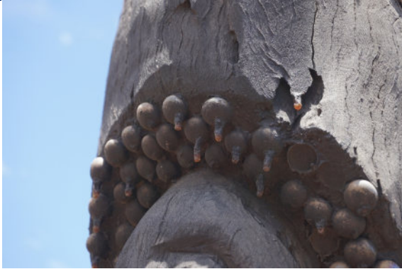
Detail 69: Detail – Pole 9, exterior, UV degradation (darkening) to wood surface, sap-like deposits (accretions) above the carved figure surrounded by glass pebbles.
