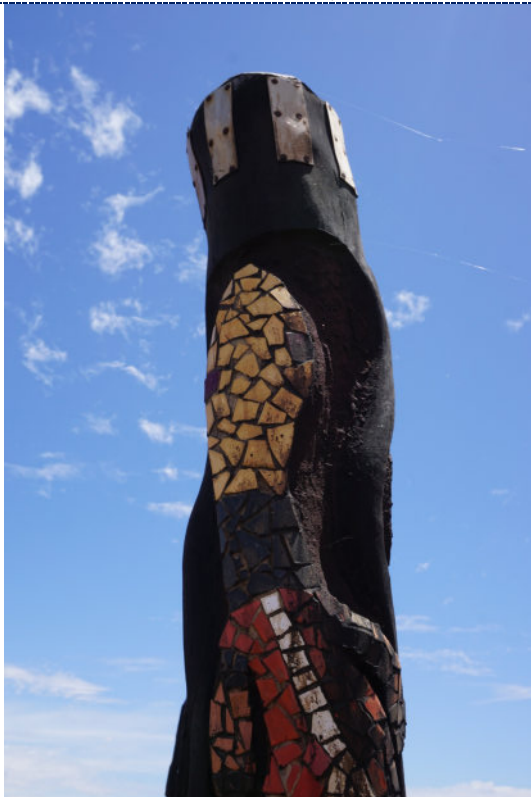
Figure 75: Detail – Pole 10, exterior, UV degradation (darkening) to wood surface, discolouration of the mosaic tiles and buildup of dirt particulate throughout.
