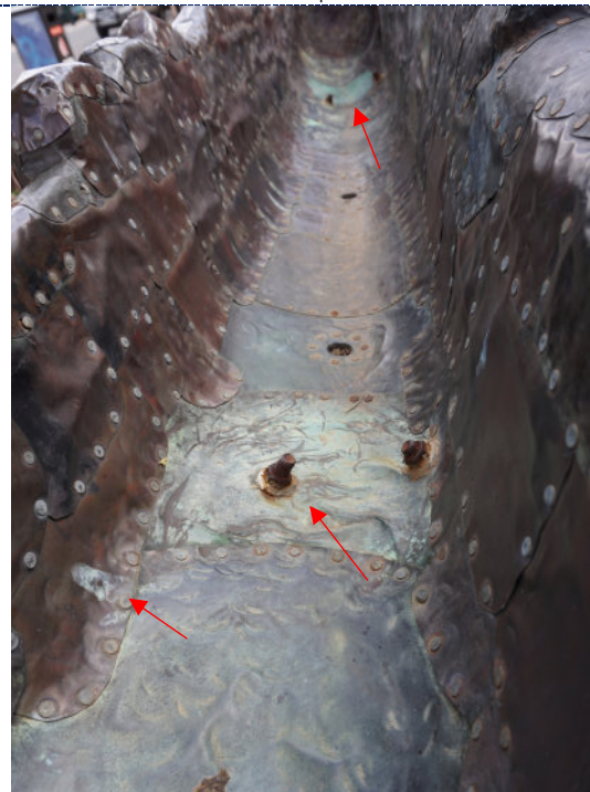
Figure 16: Detail – interior, dirt particulate, green copper corrosion in areas where water pools; corroded bolts where mounts are attached; bird excrement.
