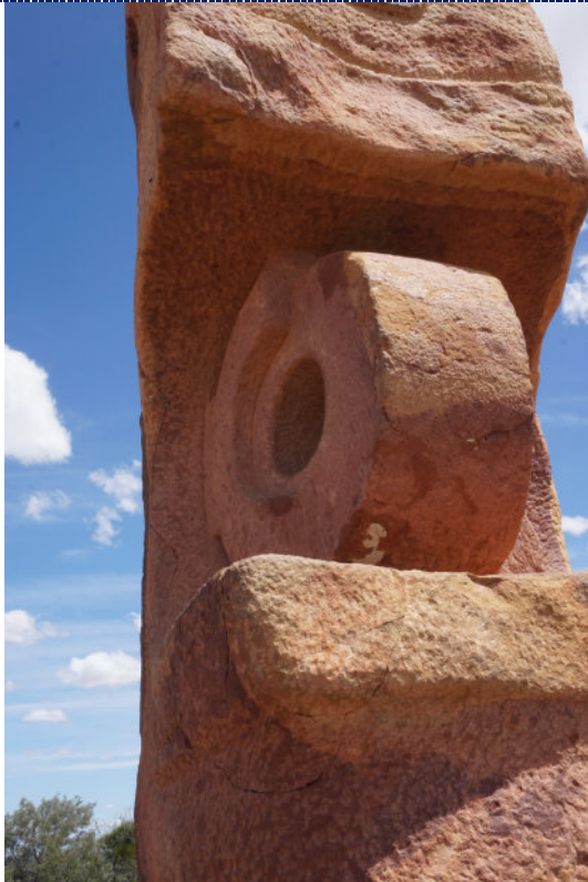
Figure 11: Detail – previous repair.
