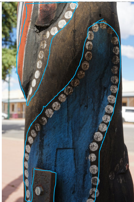
Figure 121: Detail – Pole #2003.0026, Reconciliation , exterior, UV degradation (darkening) to wood surface throughout. The painted areas are also faded and lost (highlighted in blue), which is consistent with UV degradation and display outdoors.
