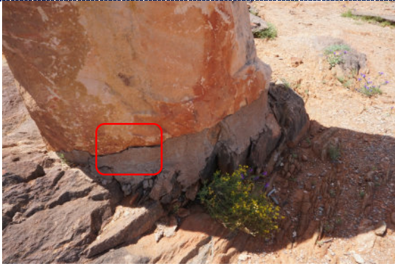
Figure 5: Detail – lifting and separation of mortar join.
