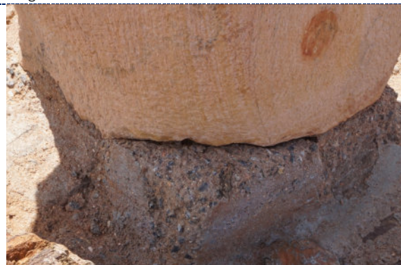
Figure 16: Detail – concrete base.
