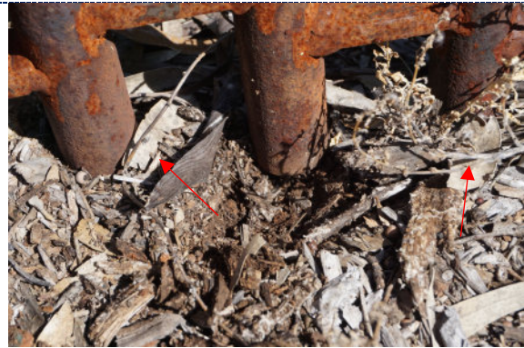
Figure 14: dirt particulate; surface flash rusting at new welds created during manufacture of artwork; biomatter collecting around the base of the work.
