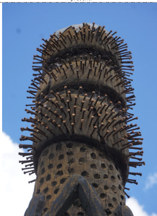
Figure 18: Detail – Pole #2003.0017 Reconciliation , exterior, corroded iron nails and metal structural components, UV degradation (darkening) to wood surface, extensive losses to painted surfaces, and extensive cracks along the grain of the wood.
