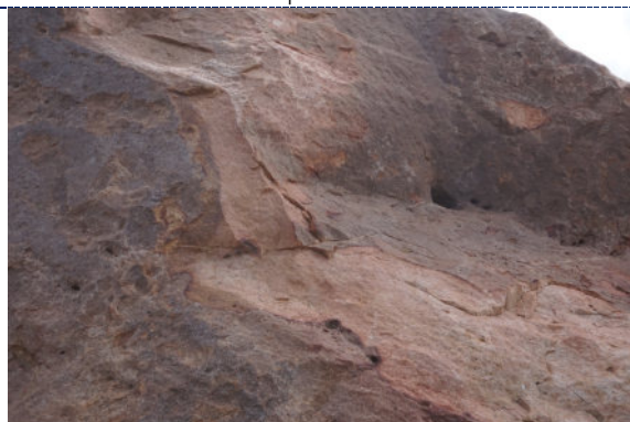
Figure 13: Detail – possible stone delamination.
