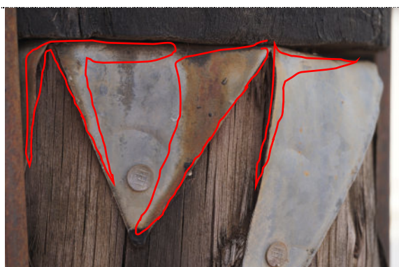
Figure 48: Detail – Pole #2003.0020 Untitled , exterior, iron corrosion and staining on the metal components and fastenings (highlighted in red). Linear cracks noted along the grain of the wood.
