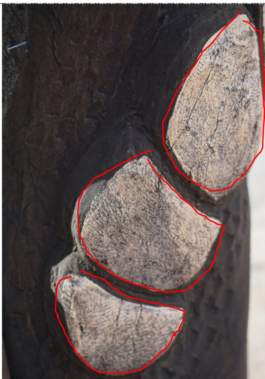
Figure 50: Detail – Pole #2003.0020 Untitled , exterior, UV degradation (darkening) to wood surface throughout. Linear cracks noted along the grain of the wood. Discolouration, losses and fading to the white painted decorative elements (highlighted in red).
