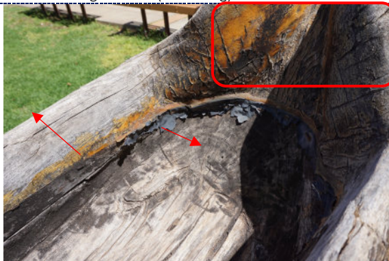
Figure 11: Detail – interior, degraded and peeling varnish, UV degradation (darkening) to wood surface. Interior poly propylene liner, silicon sealant and iron staples heavily degraded.
