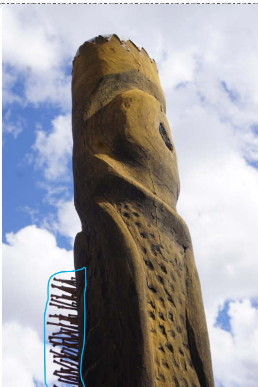
Figure 66: Detail – Pole #2003.0021 Untitled , exterior, UV degradation (darkening) to wood surface throughout. Iron corrosion on nails affixed to the timber pole (highlighted in blue).
