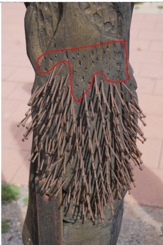
Figure 60: Detail – Pole #2003.0021 Untitled , exterior, UV degradation (darkening) to wood surface throughout. Iron corrosion on nails affixed to the timber pole. Missing iron nails are also noted on the exterior sides of the pole (highlighted in red).
