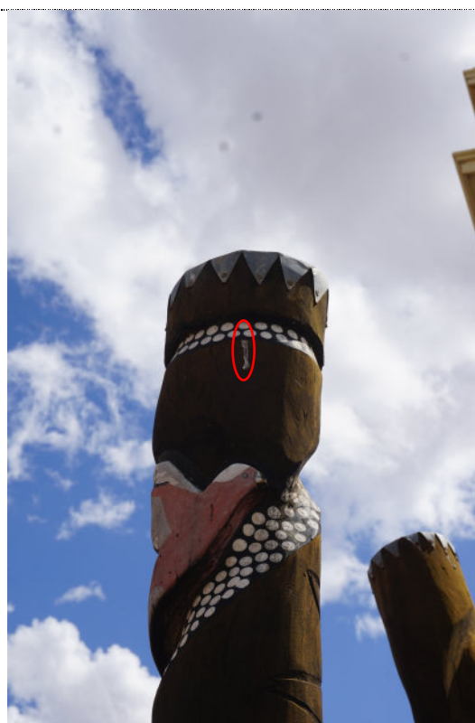
Figure 41: Detail – Pole #2003.0019 Galahs , exterior, UV degradation (darkening) to wood surface throughout. Surface dirt and insect debris noted throughout, including the presence of bird excrement (highlighted in red).
