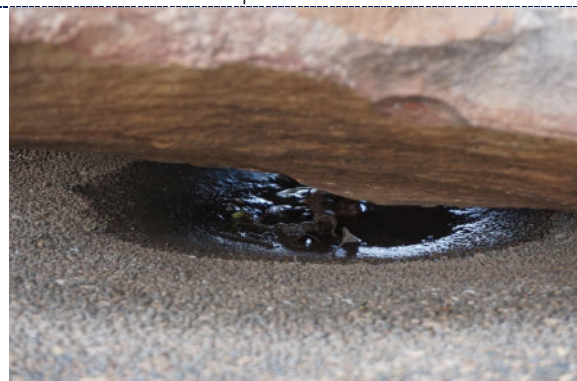
Figure 24: Detail – Component 3 – pooling water and biomatter.
