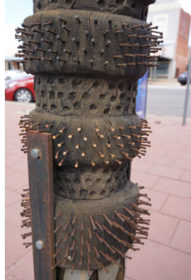
Figure 10: Detail – Pole #2003.0017 Reconciliation , proper right exterior, corroded iron nails, degraded varnish and UV degradation (darkening) to wood surface.
