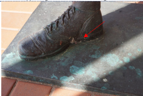
Figure 7: Detail – corrosion product, possibly stemming from acidic dog urine; dirt particulate, spider webs, bird excrement.
