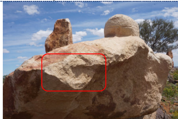
Figure 16: Detail – possible stone delamination.
