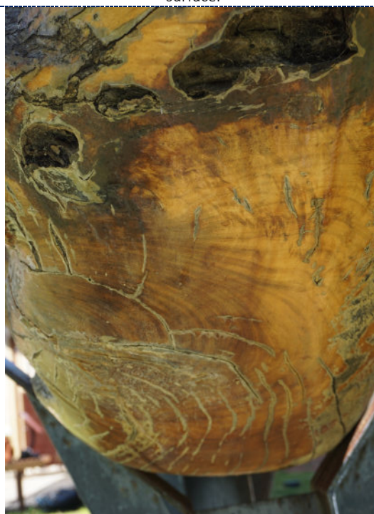
Figure 18: Detail – exterior-bottom, degraded and peeling varnish.
