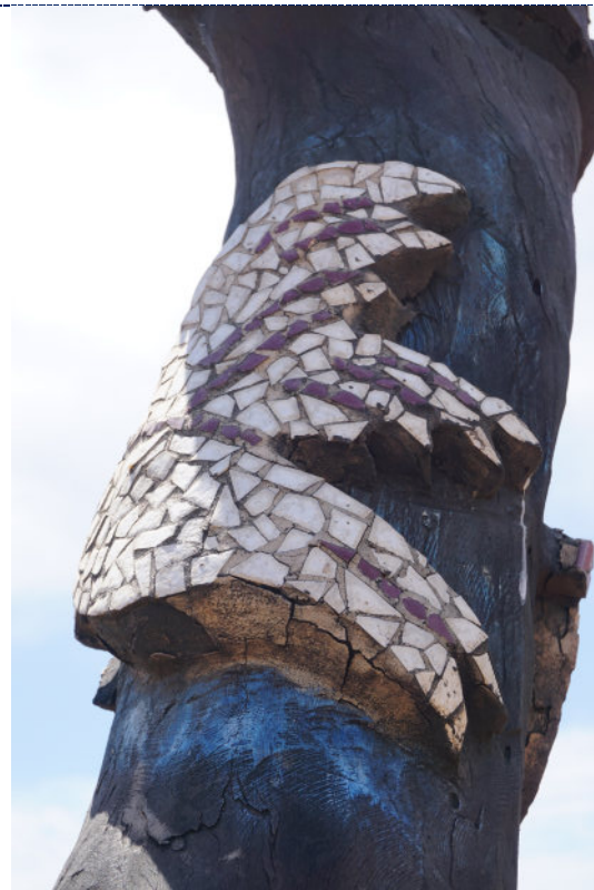
Figure 58: Detail – Pole 8, exterior, UV degradation (darkening) to wood surface, extensive losses to painted surfaces and degradation to the binder securing the mosaic tiles in place.
