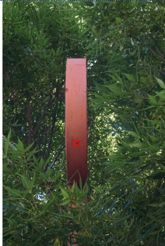
Figure 10: Detail – small hole, inherent to fabrication.
