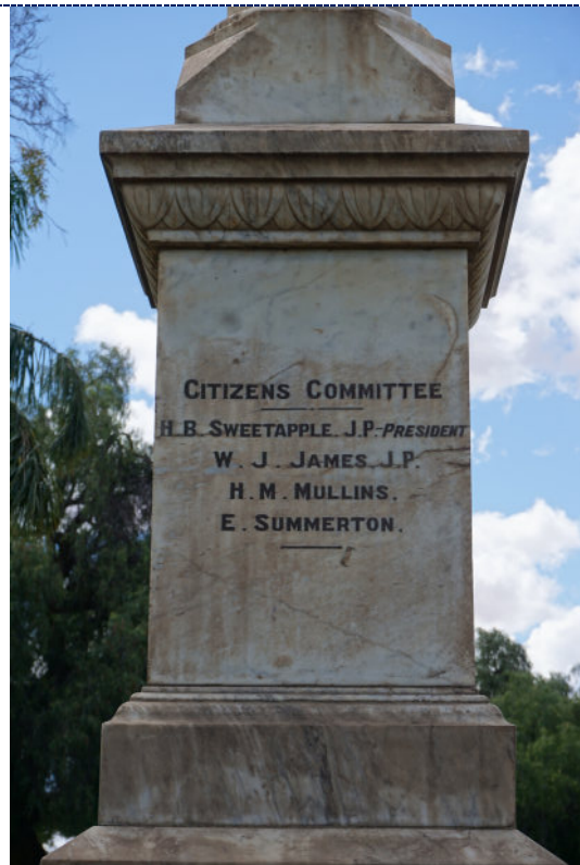
Figure 8: Detail – proper right, dirt particulate and stone discolouration.
