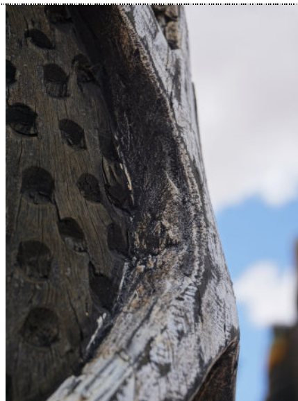
Figure 14: Detail – Pole #2003.0017 Reconciliation , exterior, UV degradation (darkening) to wood surface, and fine cracks along the grain of the wood. The surface is also covered in a layer of dirt particulate.
