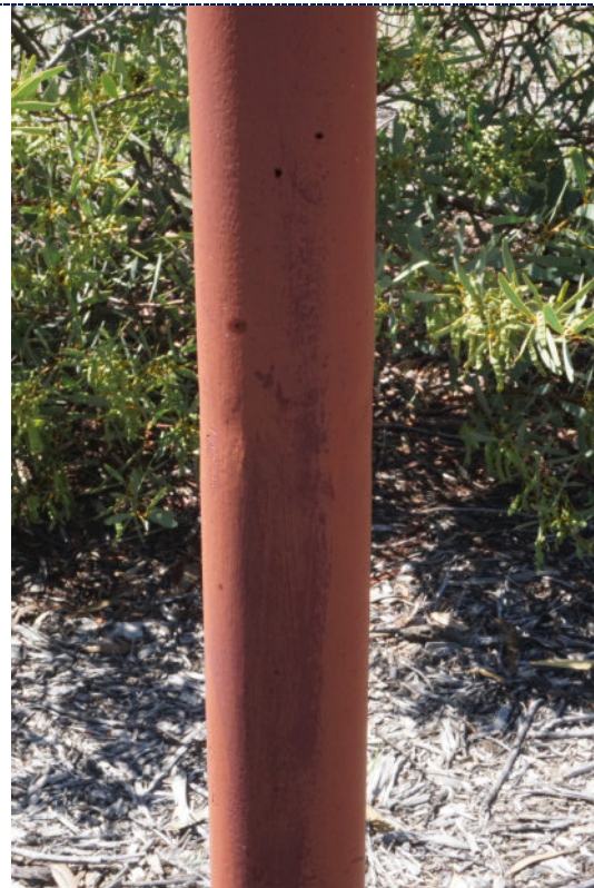
Figure 8: Detail – paint chalking, overpaint.
