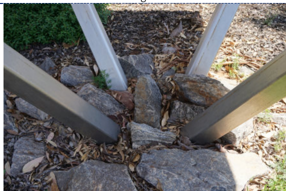
Figure 13: Detail – rocks at base for drainage and the accumulation of biomatter.
