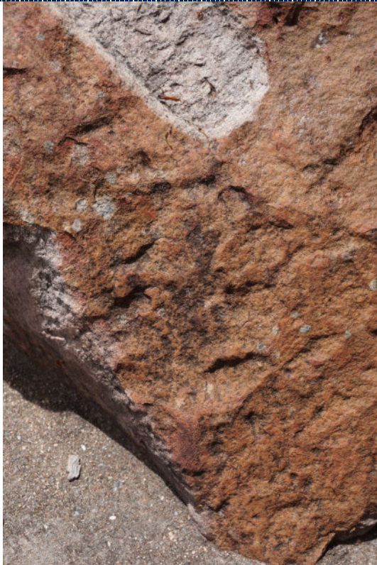
Figure 9: Detail – Component 1 – dirt particulate and spider webs.
