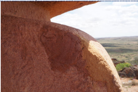
Figure 7: Detail – previous repair.
