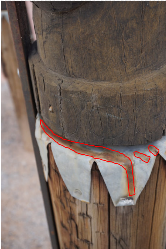
Figure 110: Detail – Pole #2003.0025, Reconciliation , exterior, iron staining to metal components (highlighted in red) and presence of corrosion products on iron nails. UV degradation (darkening) to wood surface, and multiple cracks along the grain of the wood.
