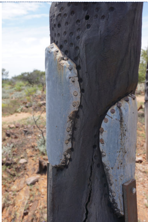
Figure 11: Detail – Pole 2, exterior, UV degradation (darkening) to wood surface, presence of ferric corrosion products on iron components and fittings. Cracks and splitting following the grain of the wood are evident throughout. Dirt particulate is present throughout.
