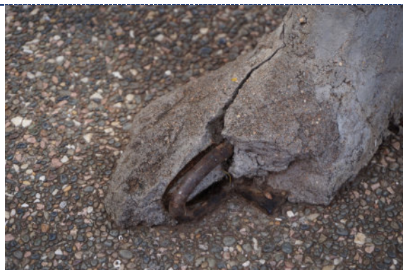
Figure 5: Figure 1 – Detail – dirt particulate, large crack and loss revealing internal iron armature.
