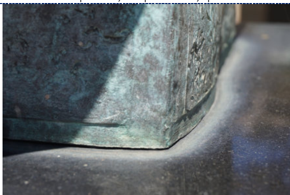
Figure 13: Detail – dirt particulate and increased copper corrosion product stemming from collected water at plinth interface.
