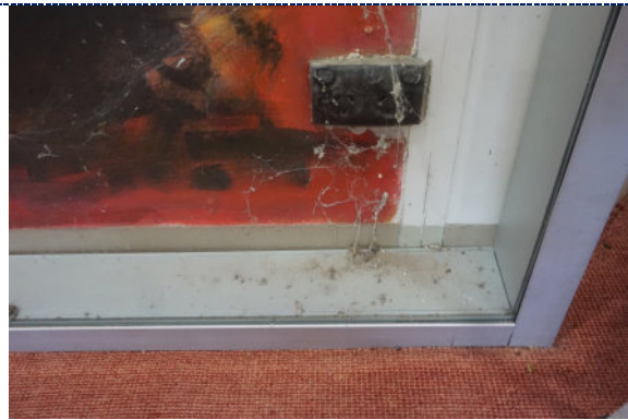
Figure 2: Section 1 – Lower proper left corner
