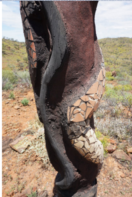
Figure 74: Detail – Pole 10, exterior, UV degradation (darkening) to wood surface, extensive losses to wood and painted surfaces and degradation to the binder securing the mosaic tiles in place.
