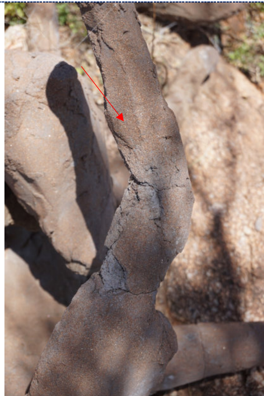
Figure 14: Detail – dirt particulate, large cracks and loss revealing internal iron armature at shoulder.
