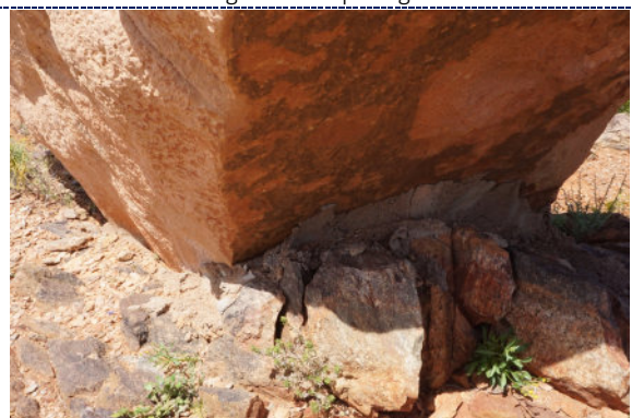
Figure 6: Detail – rear cement/concrete at base.
