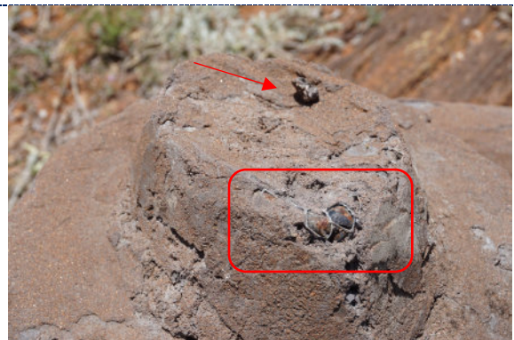
Figure 8: Detail – loss to concrete fondue revealing chicken wire and iron armature; bird excrement.
