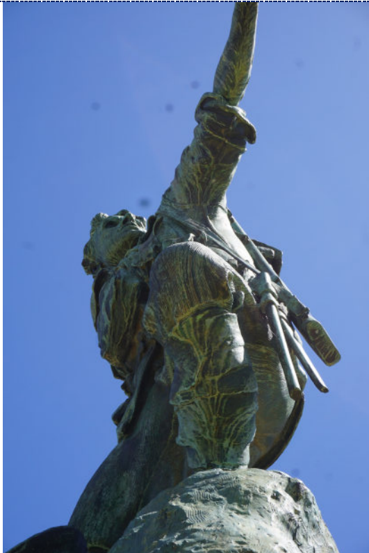
Figure 7: Detail – atmospheric pollution-driven copper corrosion product on figure.
