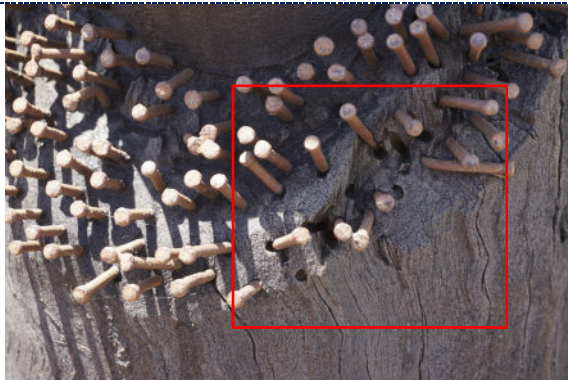
Figure 65: Detail – Pole 9, exterior, UV degradation (darkening) to wood surface, extensive losses to painted surface on carved figure's eyes. Missing nails noted below and along the periphery of the central figure (highlighted in red).
