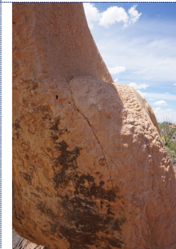
Figure 11: Detail – vertical crack with minor stone delamination.
