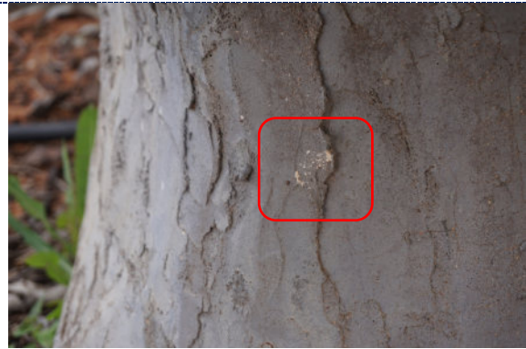
Figure 28: Figure 3 – Detail – dirt particulate, surface accretion.
