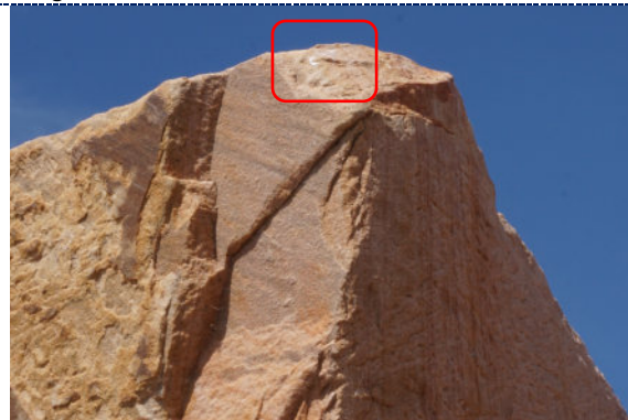
Figure 8: Details – top, stone delamination and weathering; bird excrement.
