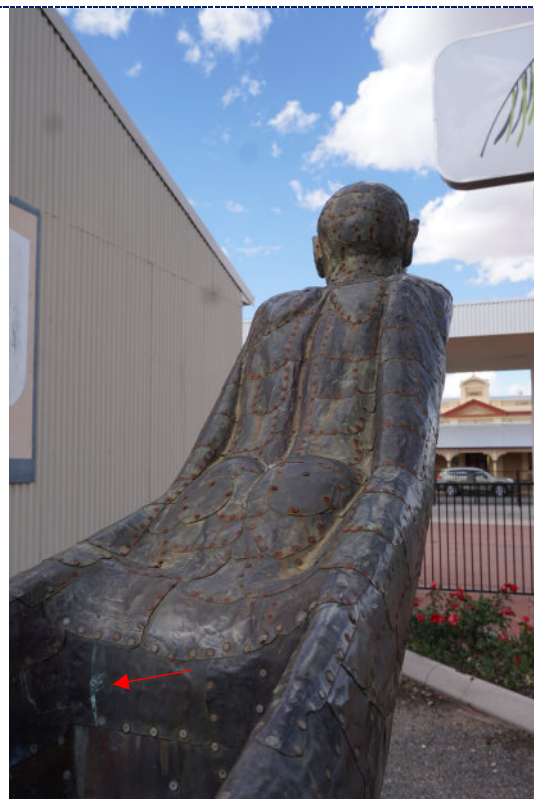
Figure 10: Detail – interior, dirt particulate, isolated surface corrosion products; corroded iron vs zinc plated nail heads; bird excrement (arrow).
