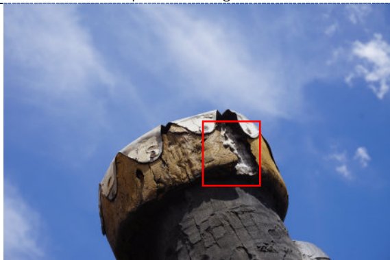
Figure 35: Detail – Pole 5, exterior, UV degradation (darkening) to wood surface, large loss to wood on exterior side of the pole's (top of pole, highlighted in red).
