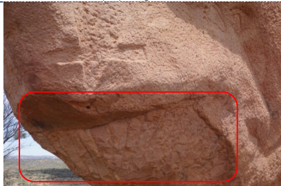
Figure 11: Detail – horizontal crack under lip of the object.
