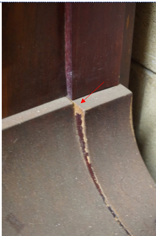
Figure 9: Detail – dirt particulate; loss to surface lacquer.
