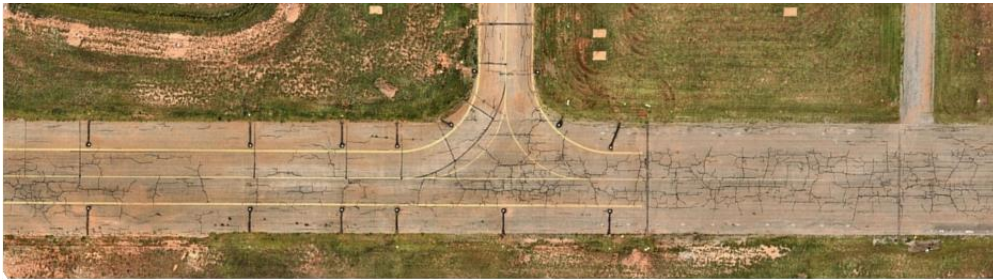
Figure 13: Taxiway Bravo Potholes
