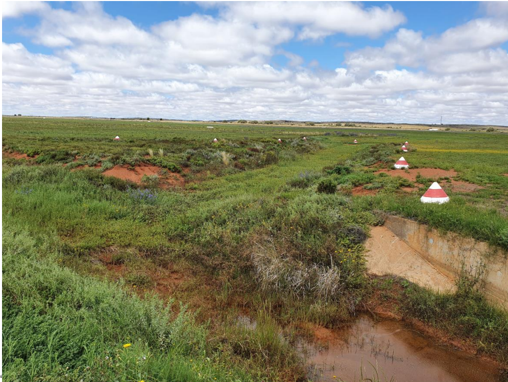
Figure 26: View of typical stormwater drain
