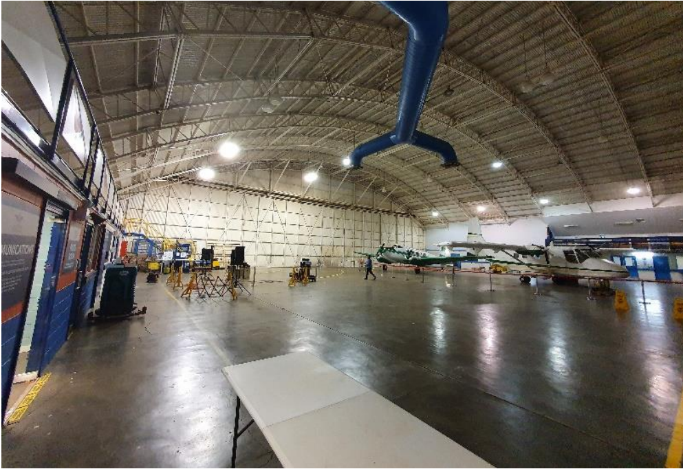
Figure 48: Internal View of Hangar Conversion
