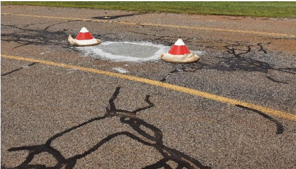
Figure 13: Taxiway Bravo Potholes
