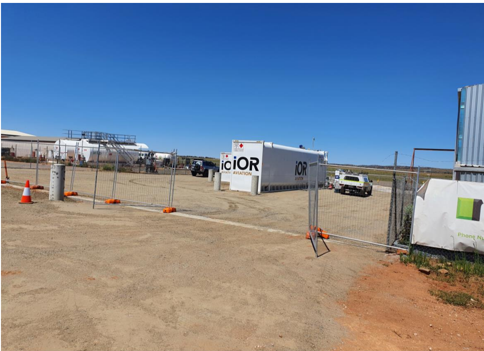
Figure 53: Viva Fuel Facility under construction
