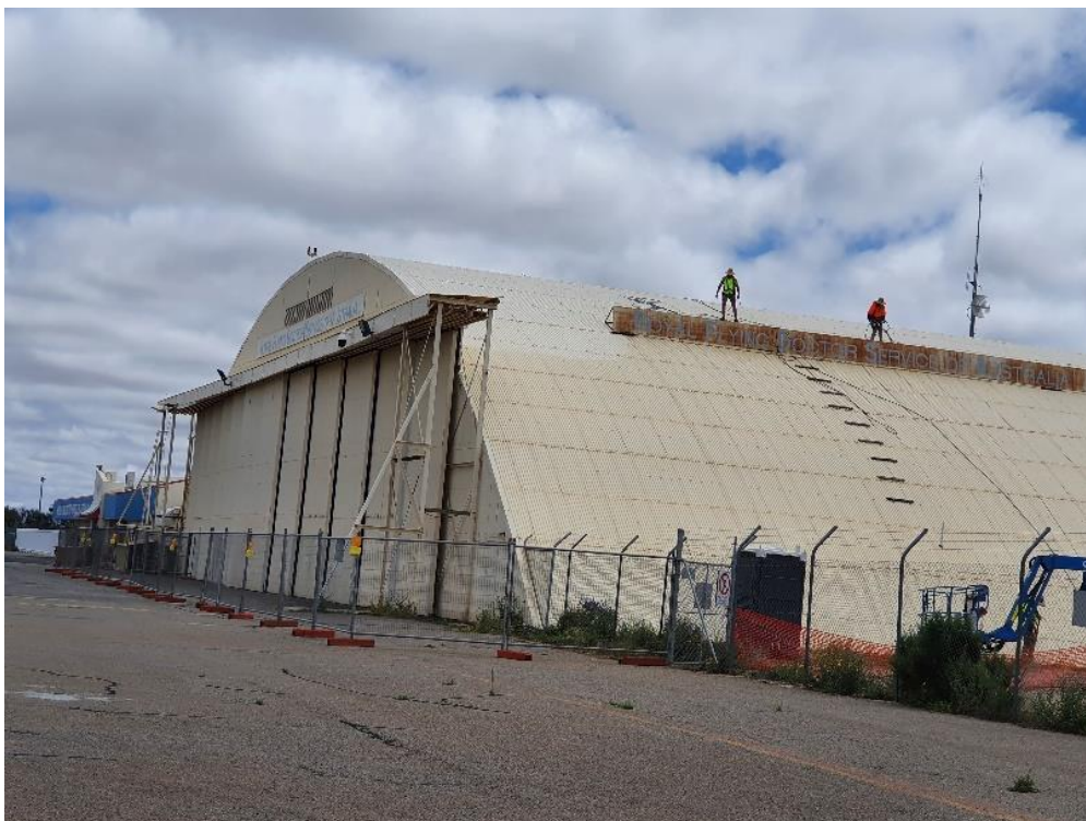
Figure 47: Old RFDS Hangar being converted to Visitors Centre
