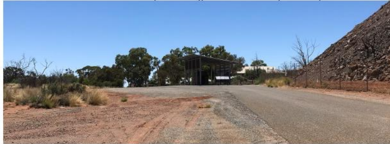
View of BHP chimney area - also part of precinct
