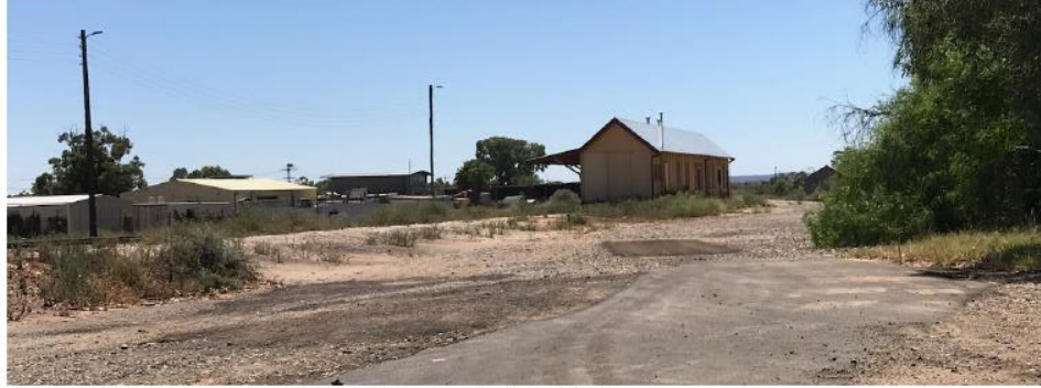
The Old Railway station surrounds - note poor condition of road
