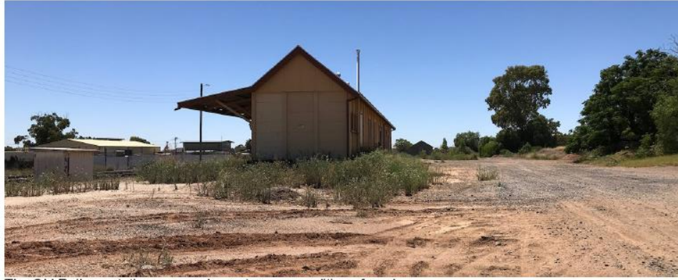
The Old Railway station surrounds - note poor condition of road
