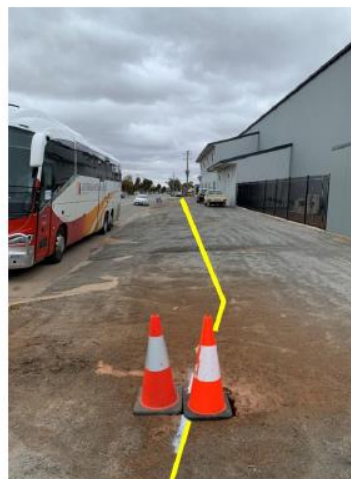
Figure 4: Delineated pipe alignment
