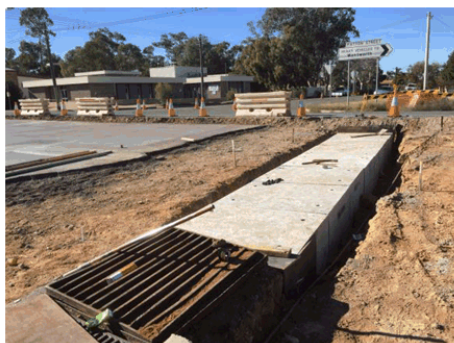
After – newly installed box culverts
