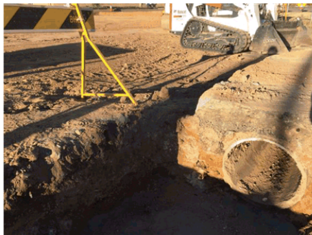
Before – aged stormwater pipes
