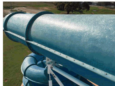
Broken Hill's extreme heat caused deterioration to the slide
