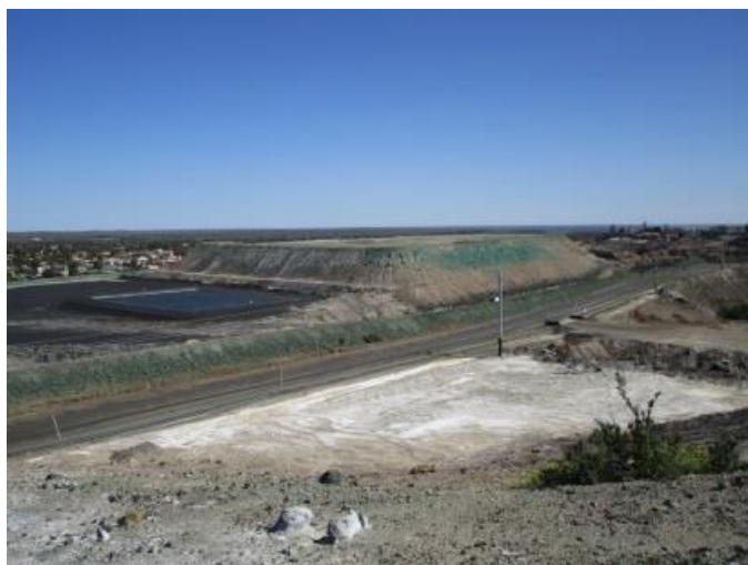
Image of a dust suppression chemical application, where a green dye is added to a solution on PVA glue which is used as a crusting agent
