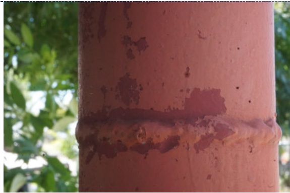
Figure 6: Detail – paint chalking, flaking paint loss with overpaint.
