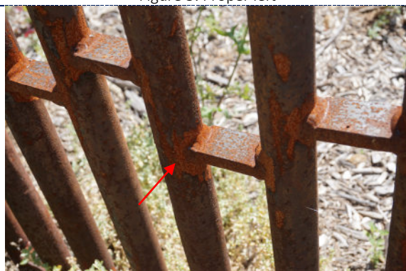
Figure 5: Detail – dirt particulate; surface flash rusting at new welds created during manufacture of artwork.
