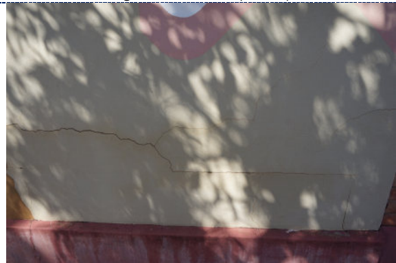
Figure 4: Detail – surface cracks and deformation to the mortar; chalking (UV degradation) and fading of the paint; staining to the exterior of the cracks.
