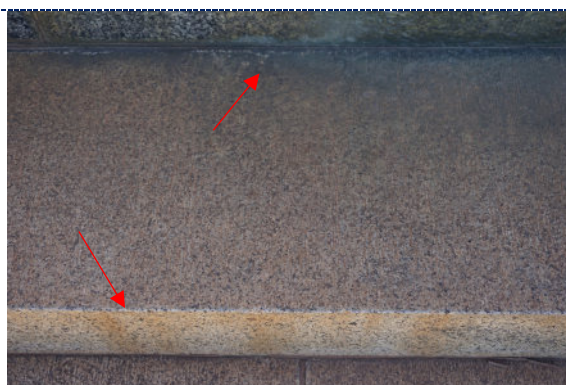
Figure 12: Detail – dirt particulate and copper corrosion product staining to granite stone; red staining at bottom may stem from iron corrosion elsewhere on the object.
