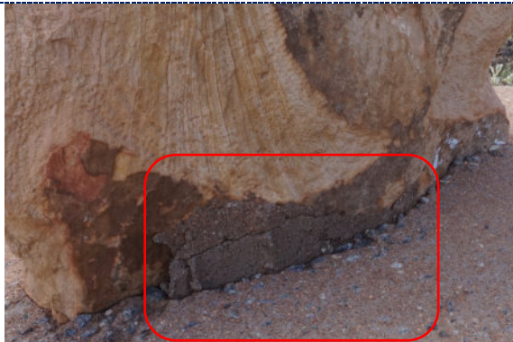
Figure 7: Detail – concrete residue on sandstone.
