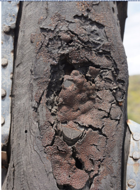
Figure 15: Detail – Pole 2, exterior, UV degradation (darkening) to wood surface, significant cracking of wood, and build-up of sap-like accretions.
