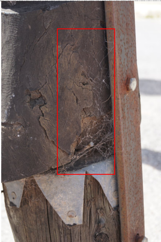
Figure 34: Detail – Pole #2003.0019 Galahs , exterior, UV degradation (darkening) to wood surface throughout. Extensive cracking and associated losses to the wood, iron corrosion noted on the iron supports and nails, and surface dirt and insect debris (spider webs, highlighted in red) noted throughout.
