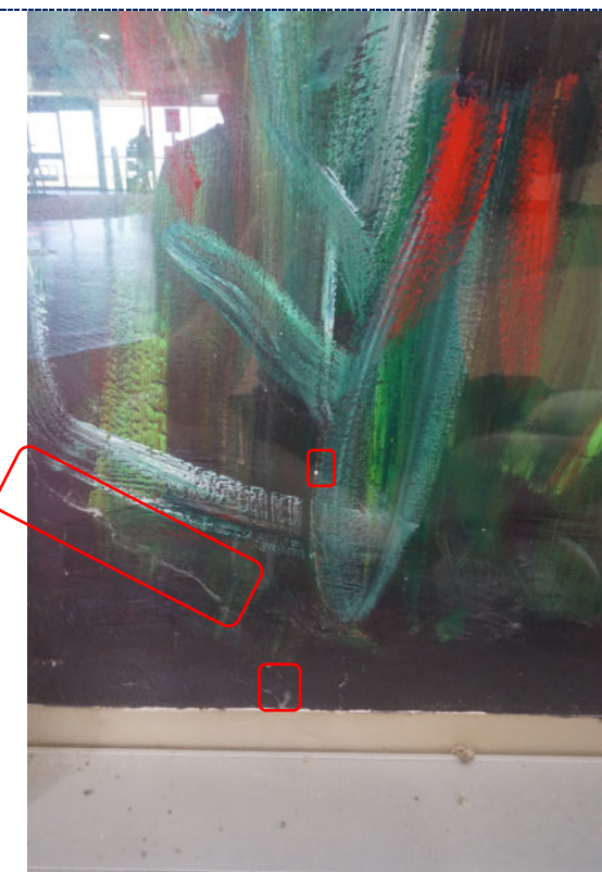
Figure 33: Section 3 – Detail – dirt particulates, spider webs and accretions.
