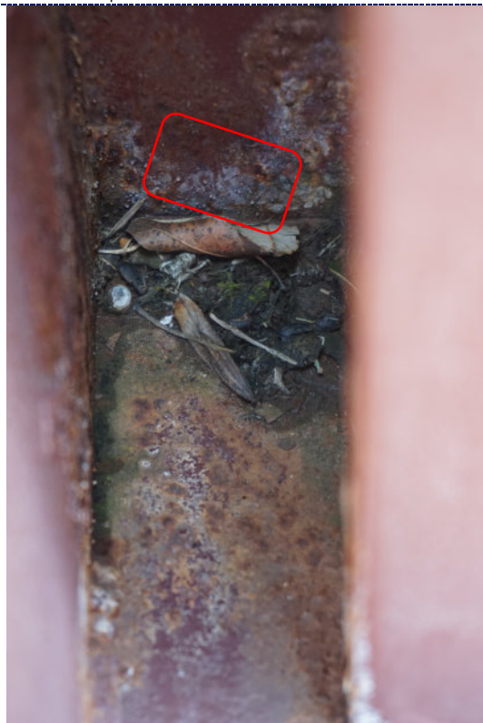
Figure 20: Detail – paint loss and corrosion to iron substrate; accumulation of dirt particulate.
