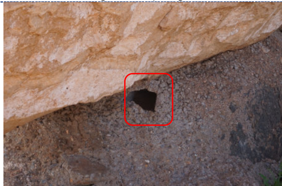
Figure 6: Detail – hole in concrete base.
