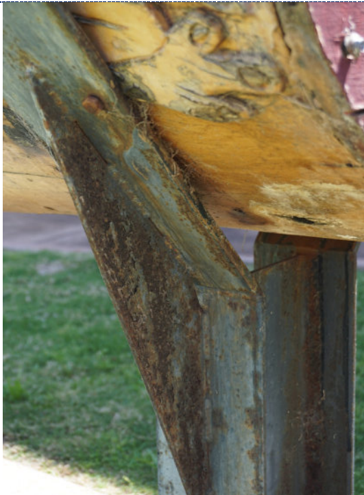
Figure 25: Detail – exterior, degraded and peeling varnish, UV degradation (darkening) to wood surface. Corrosion on mount.
