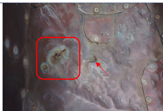
Figure 18: Detail – exterior, corrosion perforating copper plate; minor corrosion to zinc nail heads.
