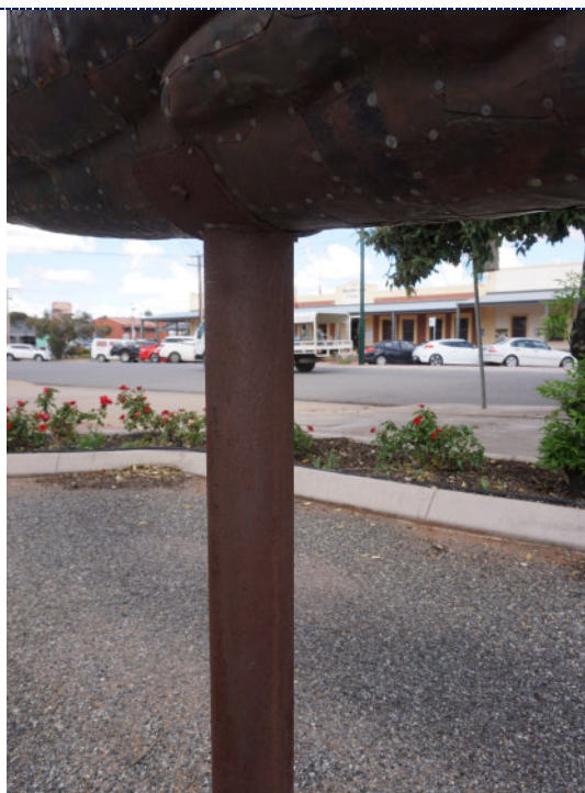
Figure 27: Detail – exterior, surface corrosion on iron mount.
