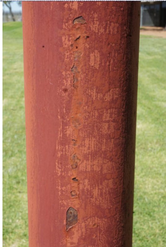
Figure 8: Detail – paint chalking, flaking paint loss with overpaint; corrosion in areas of paint loss.
