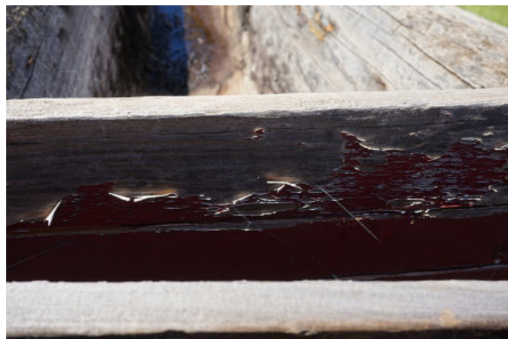
Figure 21: Detail – exterior, degraded and peeling maroon paint, UV degradation (darkening) to wood surface.
