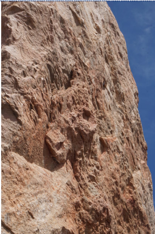
Figure 7: Detail – minor stone delamination.
