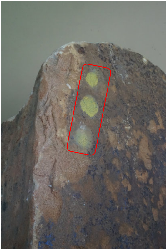
Figure 11: Detail – 3 x yellow accretion deposits.
