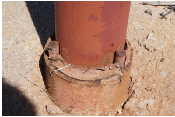
Figure 6: Detail – paint chalking, flaking paint loss with overpaint; corrosion in areas of paint loss; previous repairs (putty/silicone at base).
