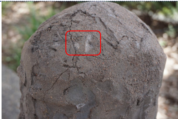
Figure 9: Figure 1 – Detail – dirt particulate, surface cracks and surface abrasion.
