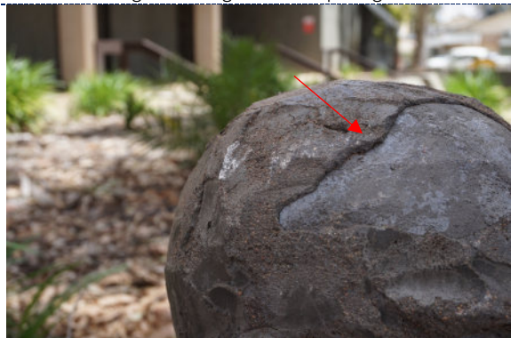
Figure 18: Figure 2 – Detail – dirt particulate, surface abrasion, surface accretion, loss to layer of cement fondue (arrow).
