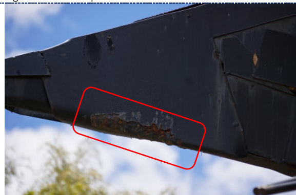
Figure 10: Detail – paint loss and corrosion to iron substrate.
