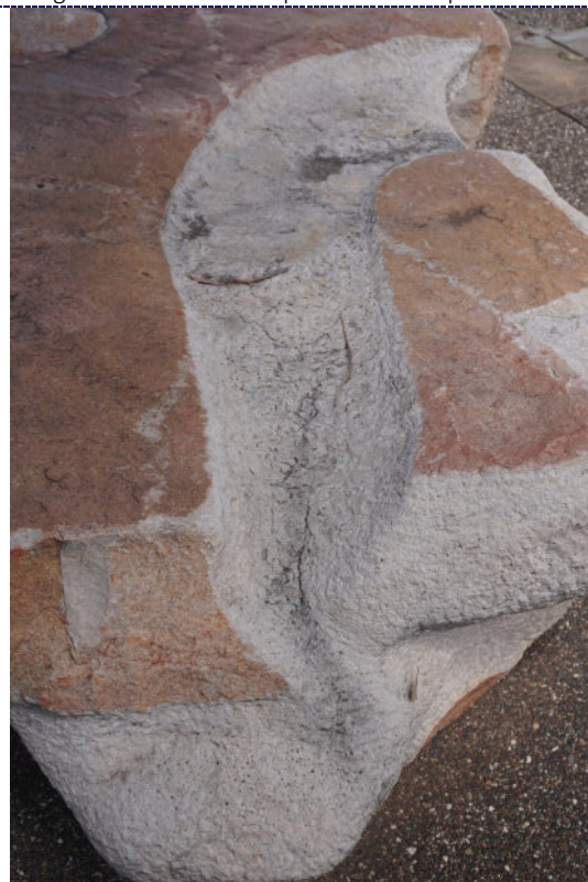
Figure 31: Detail – Component 1 – dirt particulate from water pooling.
