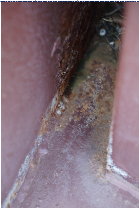
Figure 19: Detail – paint loss and corrosion to iron substrate; accumulation of dirt particulate.
