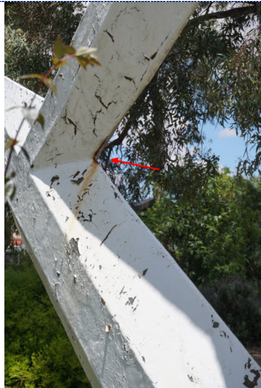
Figure 12: Detail – dirt particulate and significant surface paint loss and crazing; iron corrosion product staining (arrow).
