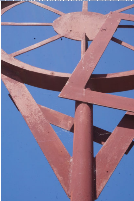
Figure 7: Detail – paint chalking, overpaint; spider webs, bird excrement.
