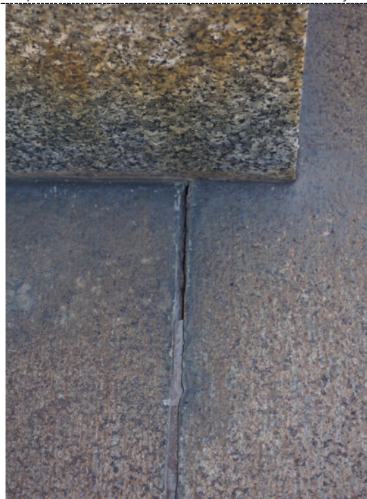
Figure 14: Detail – dirt particulate, red staining (possibly iron corrosion product) and loss to mortar pointing.
