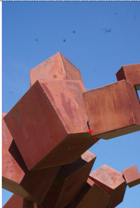
Figure 8: Detail – paint chalking, flaking paint loss with overpaint; dirt particulate and spider webs. The two shades of red paint suggest the surface was repainted.
