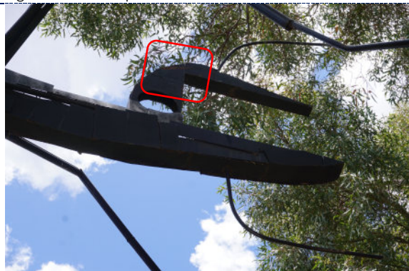
Figure 7: Detail – paint loss and corrosion to iron substrate.
