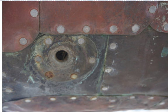
Figure 30: Detail – exterior, dirt particulate, spider webs; corrosion to zinc nail heads; biomatter clogging drains.
