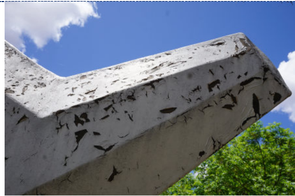
Figure 10: Detail – dirt particulate and significant surface paint loss and crazing.
