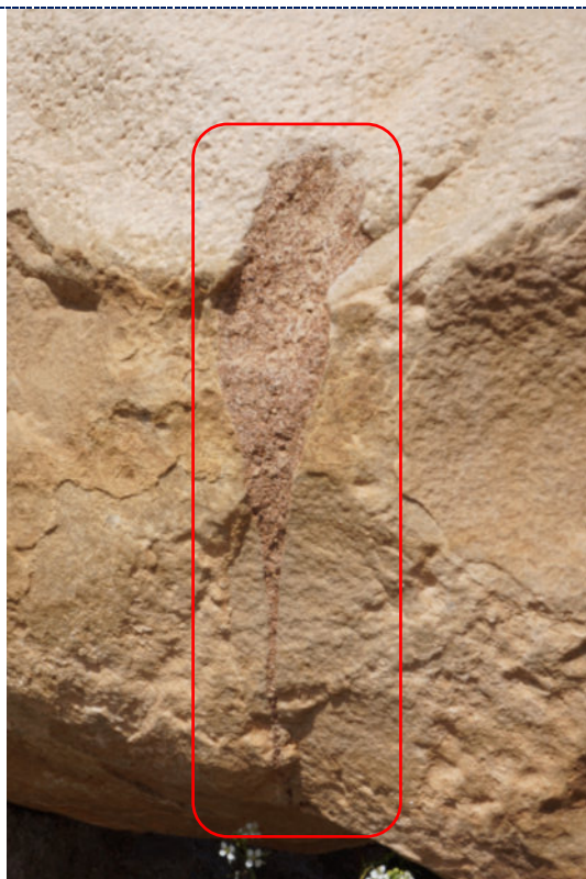
Figure 11: Detail – mortar fill.
