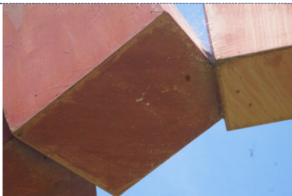
Figure 9: Detail – paint chalking, flaking paint loss with overpaint; dirt particulate and spider webs.
