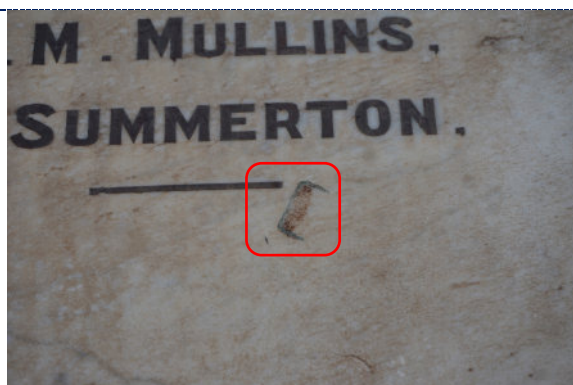
Figure 15: Detail – dirt particulate, surface abrasion with paint transfer.
