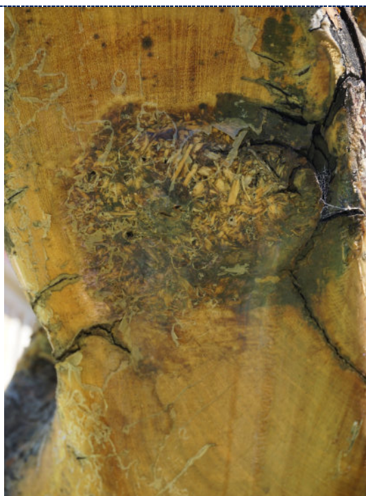
Figure 17: Detail – exterior-bottom, degraded and peeling varnish.
