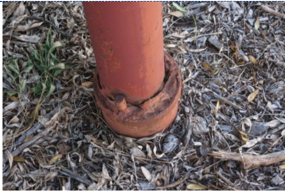
Figure 5: Detail – base plinth, paint chalking, flaking paint loss with corrosion and putty deterioration.
