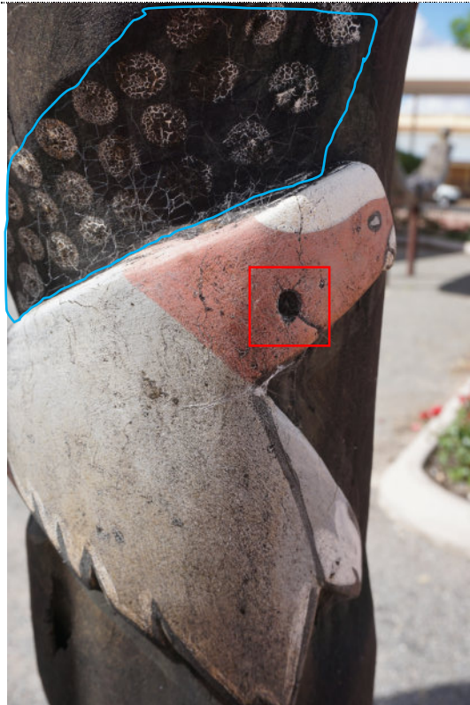
Figure 35: Detail – Pole #2003.0019 Galahs , exterior, UV degradation (darkening) to wood surface throughout. Surface dirt and insect debris noted throughout. Fading noted to the painted surfaces, particularly the painted galahs and the surrounding dots (highlighted in blue). Missing nail noted to the neck of the carved galah (highlighted in red).
