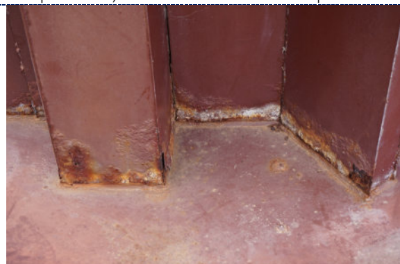
Figure 16: Detail – paint fading and degradation; dirt particulate and surface accretions (white); iron corrosion.
