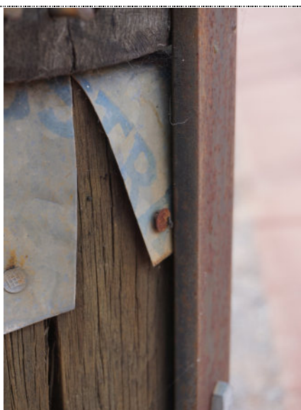
Figure 13: Detail – Pole #2003.0017 Reconciliation , exterior, corroded iron nails and metal components, UV degradation (darkening) to wood surface, and fine cracks along the grain of the wood.
