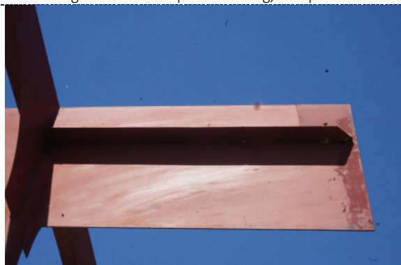
Figure 10: Detail – paint chalking, overpaint.
