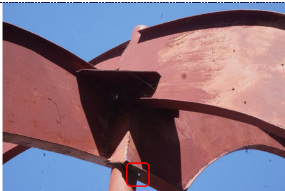
Figure 13: Detail – chalking paint, flaking paint loss, abrasions and corrosion; overpaint; corrosion resulting in perforation of the substrate (small hole).
