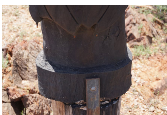
Detail 84: Detail – Pole 11, exterior, UV degradation (darkening) to wood surface, sap-like deposits (accretions) (highlighted in red). Iron corrosion products present on metal components, including the iron nails.
