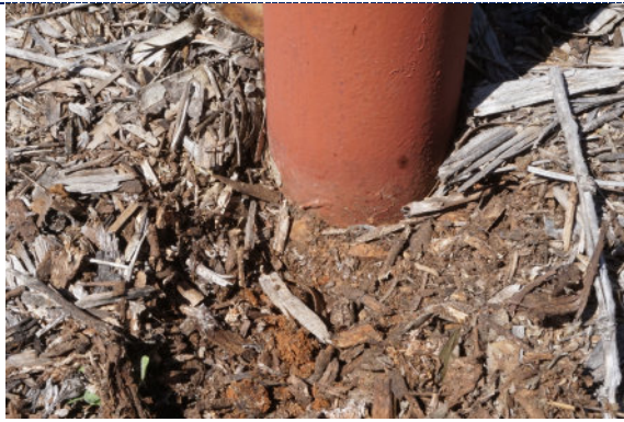
Figure 5: Detail – accumulation of biomatter at base.
