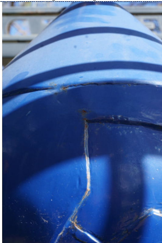
Figure 8: Detail – blanching of blue paint layer, appearing as white hazy bloom on upper section of 'drop' component. Minor losses and areas of corrosion also visible.
