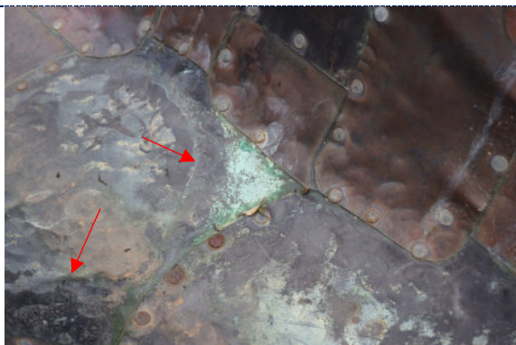
Figure 23: Detail – interior, dirt particulate, green copper corrosion in areas where water pools.
