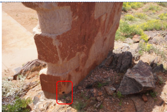
Figure 5: Detail – hole at base; minor surface abrasions.
