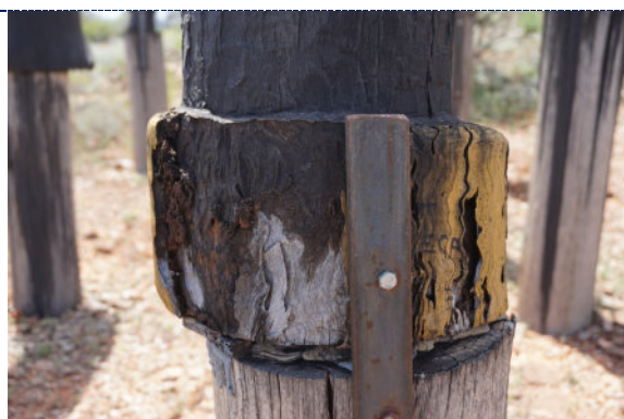
Figure 27: Detail – Pole 4, exterior, UV degradation (darkening) to wood surface, losses to wood likely associated with past insect activity, iron corrosion on metal support brackets. Dirt particulate is present throughout.
