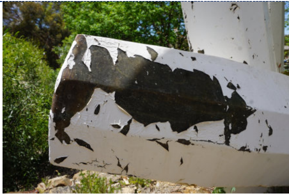
Figure 9: Detail – dirt particulate and significant surface paint loss and crazing.
