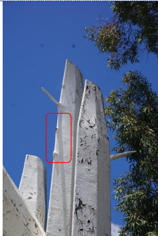
Figure 18: Detail – dirt particulate and significant surface paint loss and crazing; missing spikes.
