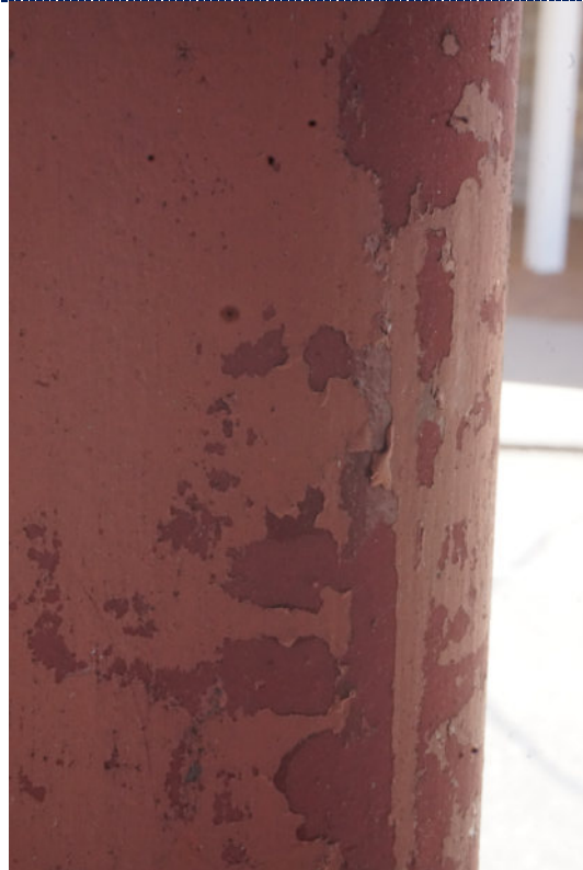
Figure 10: Detail – paint chalking, flaking, overpaint.
