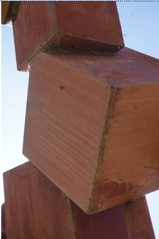
Figure 7: Detail – paint chalking, flaking paint loss with overpaint; dirt particulate and spider webs.
