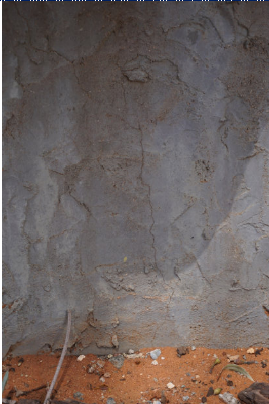
Figure 35: Figure 3 – Detail – dirt particulate, surface cracks.
