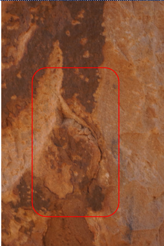
Figure 13: Detail – minor stone delamination.
