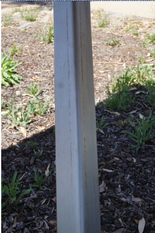
Figure 7: Detail – linear scratch and iron corrosion product.
