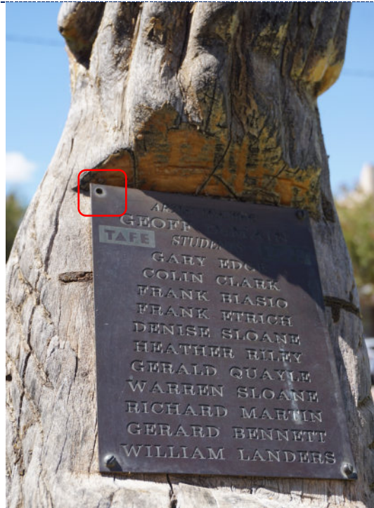
Figure 26: Detail – copper alloy plaque with bird excrement and one screw missing.
