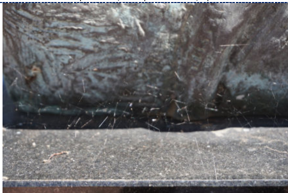
Figure 11: Detail – atmospheric pollution-driven copper corrosion product, dirt particulate, spider webs.
