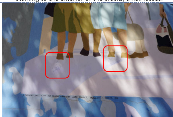
Figure 20: Detail – surface cracks and deformation to the mortar; chalking (UV degradation) and fading of the paint; staining to the exterior of the cracks; inked graffiti.
