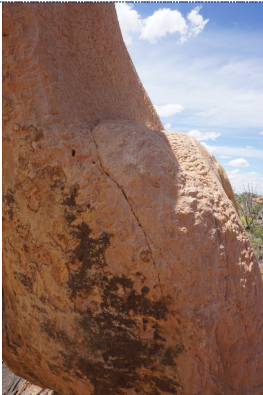
Figure 11: Detail – vertical crack with minor stone delamination.
