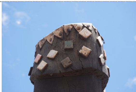
Detail 56: Detail – Pole 8, exterior, UV degradation (darkening) to wood surface, iron corrosion exhibited on metal components at top of pole. Dirt particulate present on diamond shaped tiles and throughout.
