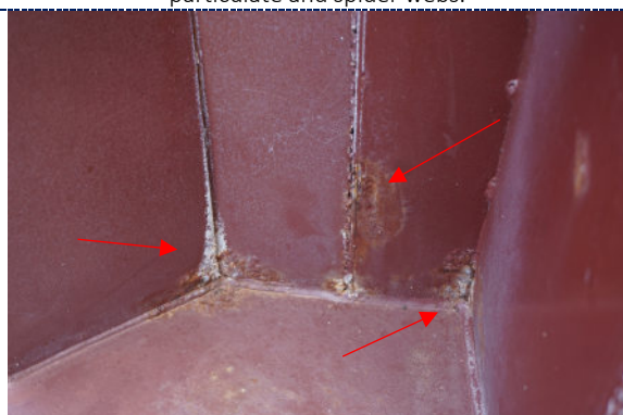
Figure 9: Detail – paint fading and degradation; dirt particulate and surface accretions (white); iron corrosion.
