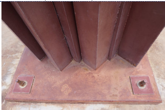
Figure 13: Detail – paint fading and degradation; dirt particulate; iron corrosion; artist's signature.
