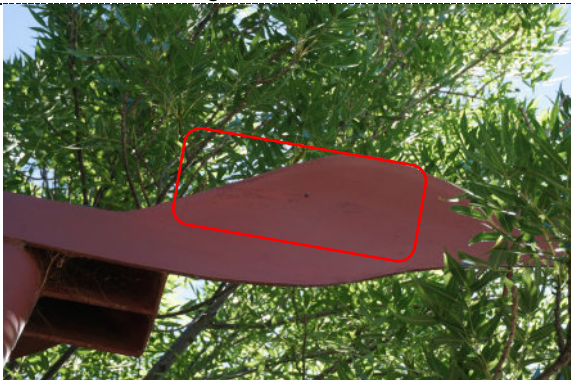
Figure 5: Detail – flaking paint loss.
