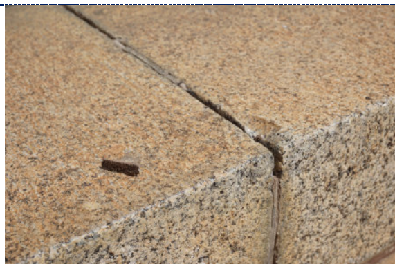
Figure 15: Detail – dirt particulate, red staining (possibly iron corrosion product) and loss to mortar pointing.
