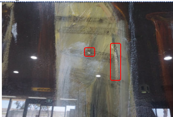
Figure 7: Section 1 – Detail – abrasions with loss.
