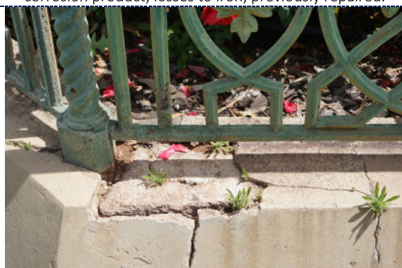
Figure 27: Detail – cracks and loss to plinth render with biogrowth; loss and degradation of green paint on cast iron fencing; iron corrosion product.
