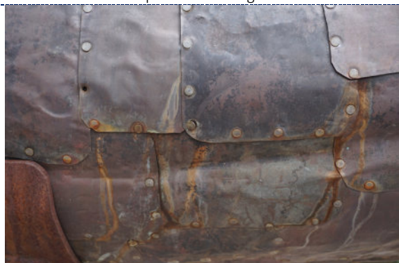
Figure 34: Detail – exterior, missing and loose nail; corroding zinc-iron nails; significant iron corrosion staining.
