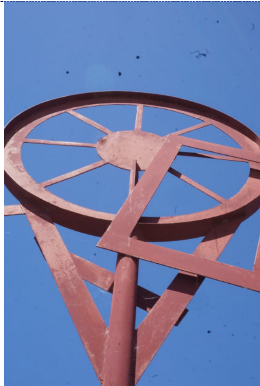
Figure 8: Detail – paint chalking, overpaint; spider webs, bird excrement.
