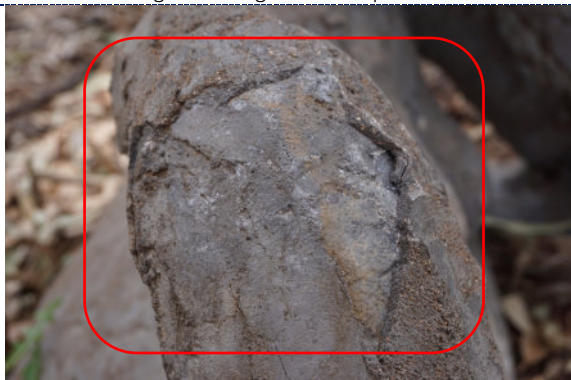
Figure 17: Figure 2 – Detail – dirt particulate, surface abrasion, loss to layer of cement fondue.
