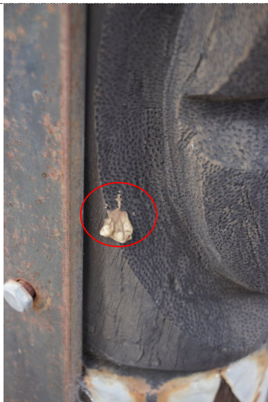
Figure 144: Detail – Pole #2003.0028, Emu and kangaroo tracks , exterior, UV degradation (darkening) to wood surface throughout. A large accretion noted on the wood surface (highlighted in red).
