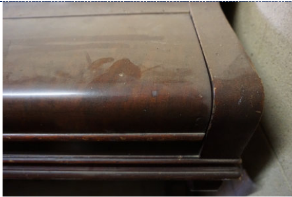
Figure 11: Detail – dirt particulate; surface accretions.
