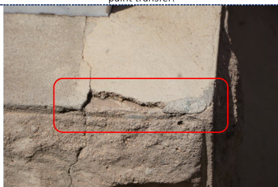
Figure 17: Detail – small cracks and loss to plinth render.
