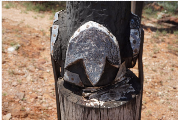
Figure 39: Detail – Pole 6, exterior, UV degradation (darkening) to wood surface, degradation of metal and presence of iron corrosion products. Dirt particulate is present throughout.
