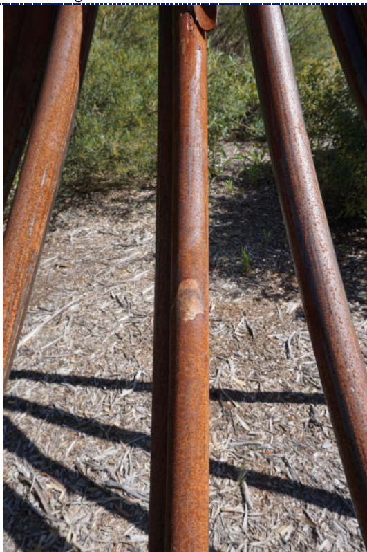
Figure 13: Detail – bird excrement; surface corrosion.
