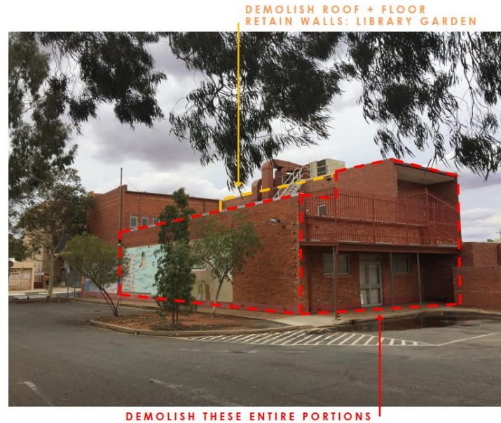
Photograph: Sections to be demolished for the new Library
