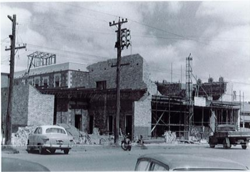
Photograph: Old Fire Station being demolished for the Library Precinct.
