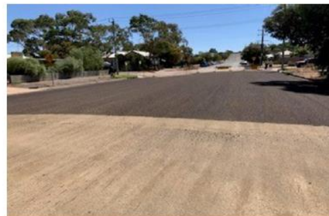
Harris Street from Burke Street to Wills Street
