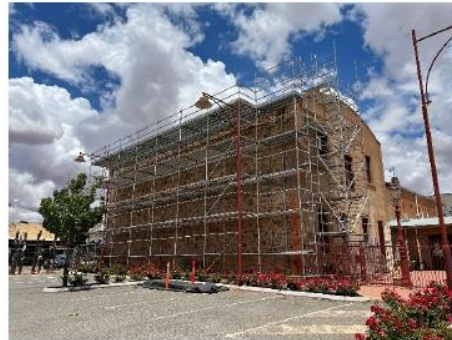
Art Gallery in preparation for roof replacement
