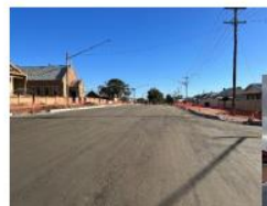
Gypsum/Pell Street Intersection looking North
