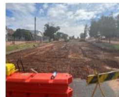
Iodide Street from Union Street looking North (during construction)
