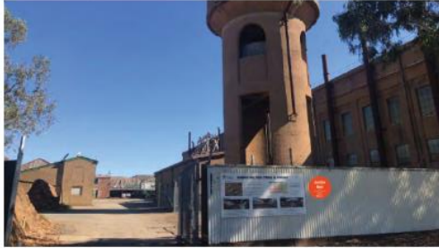
73 ● Central Power Station - 1930 (73) WALL MOUNTED ST D2.1
