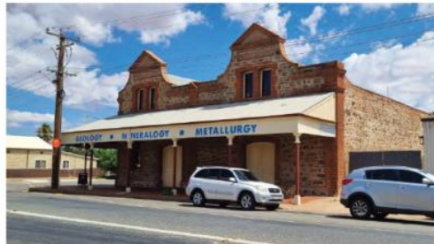
17 ● Bond Store - 1890 (17) EXISTING POST S1 D2.1
