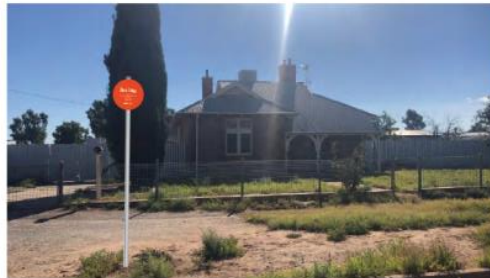
62 ● Former North Police Station - c1890 (62) S1 D2.2 LARGE FREESTANDING
