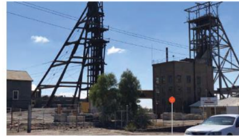
06 South Mine Headframes - 1919/1932 (96) LARGE FREESTANDING S1 D2.2
