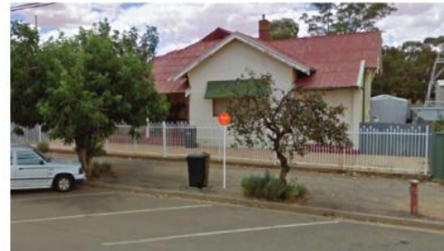
78 ● South Post Office -1898 (78) LARGE FREESTANDING ST D2.2
