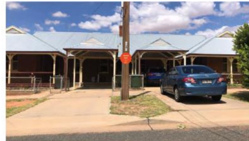
24 Former Police Barracks - 1900 (24) EXISTING POST S1 D2.1
