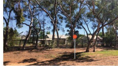
03 NBHC Mine Housing - c1950 (93) LARGE FREESTANDING S1 D2.2
