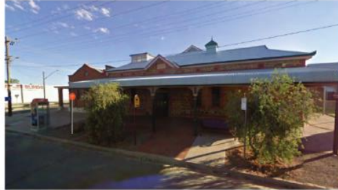
10 ● Railwaytown Post Office - 1925 (101)
