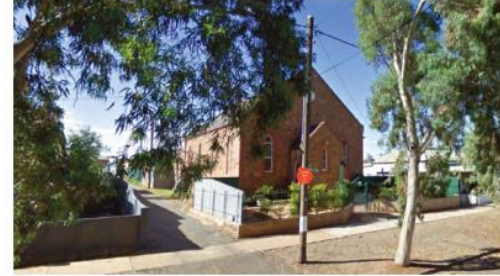
39 ● St Andrews Uniting Church - 1905 (39) EXISTING POST S1 D2.1
