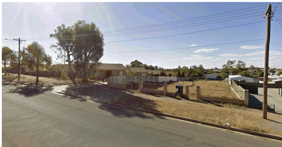
Figure 3 – 478 Cummins Street adjacent to proposed site viewed from Cummins Street.
