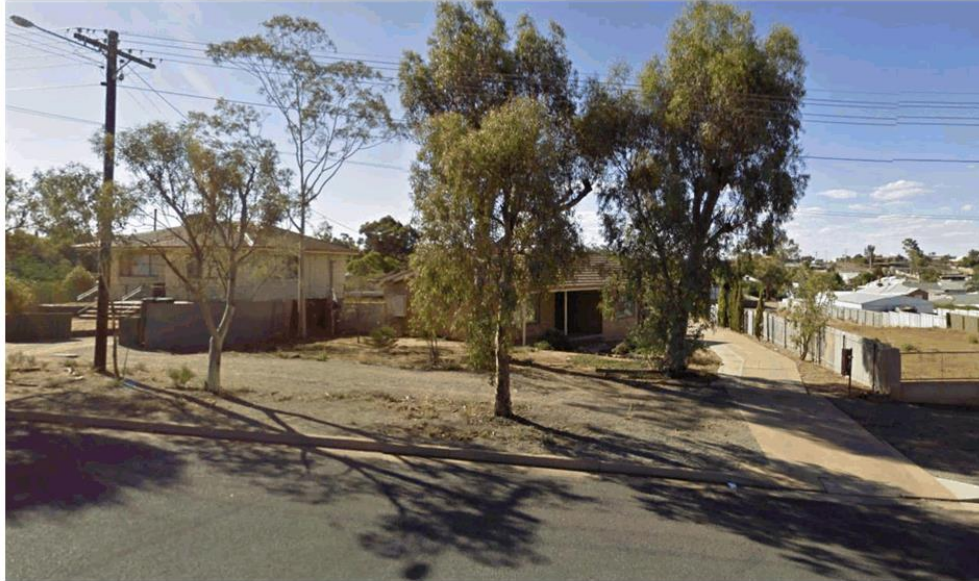
Figure 7 – 474 and 478 Cummins Street south-west of the site showing simple fenestration arrangement of a central door with windows on either side.
