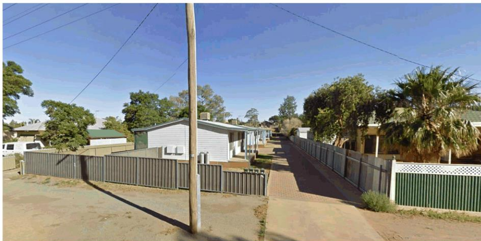
Figure 5 – 471 Wyman Street with 4 units behind the proposed site, viewed from Cummins Lane.
