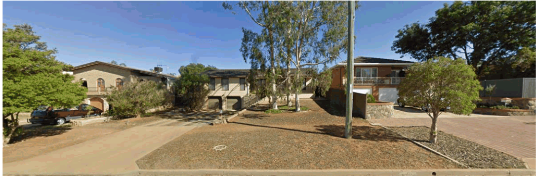
Figure 9 – 479, 481 and 483 Cummins Street - two-storey dwellings opposite to the proposed site with prominent bulk, multiple garage doors and wide driveways dominating the streetscape.
