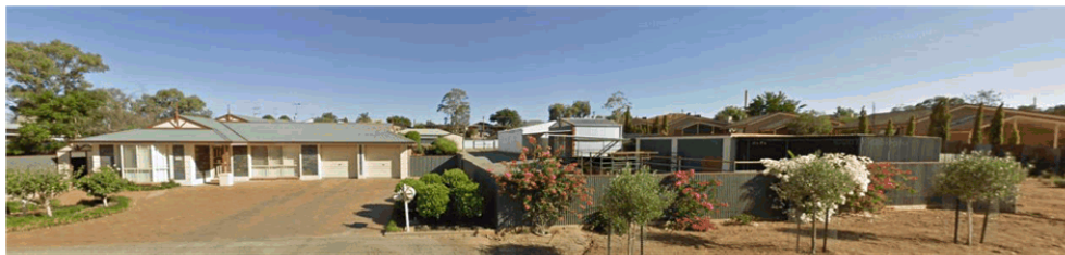
Figure 10 – 473 Cummins Lane north east to the site.
