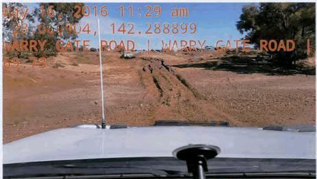
Figure 5 - Wet weather impacts cause severe road degradation
