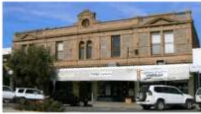
Pirie Building - Existing condition
