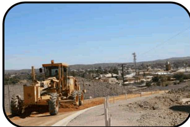
Work in progress on Federation Way
