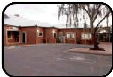
Car Park Extension
