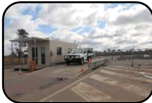
Waste Management Facility upgrades include a new weighbridge
