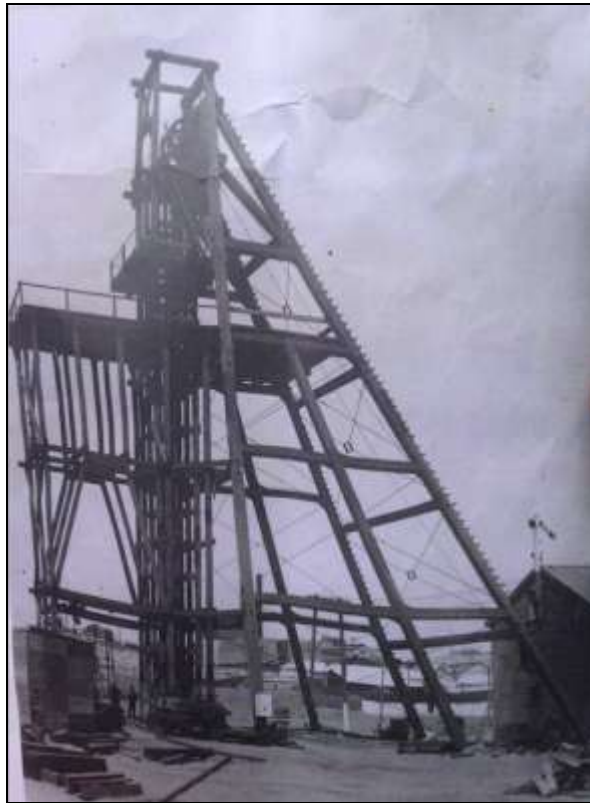
Headframe showing bracing to the north side no longer present.
